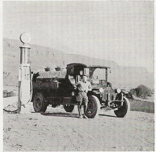
Union Oil Company tank truck making delivery of gasoline to the storage tank of the L. Romano Engineering Corporation.
