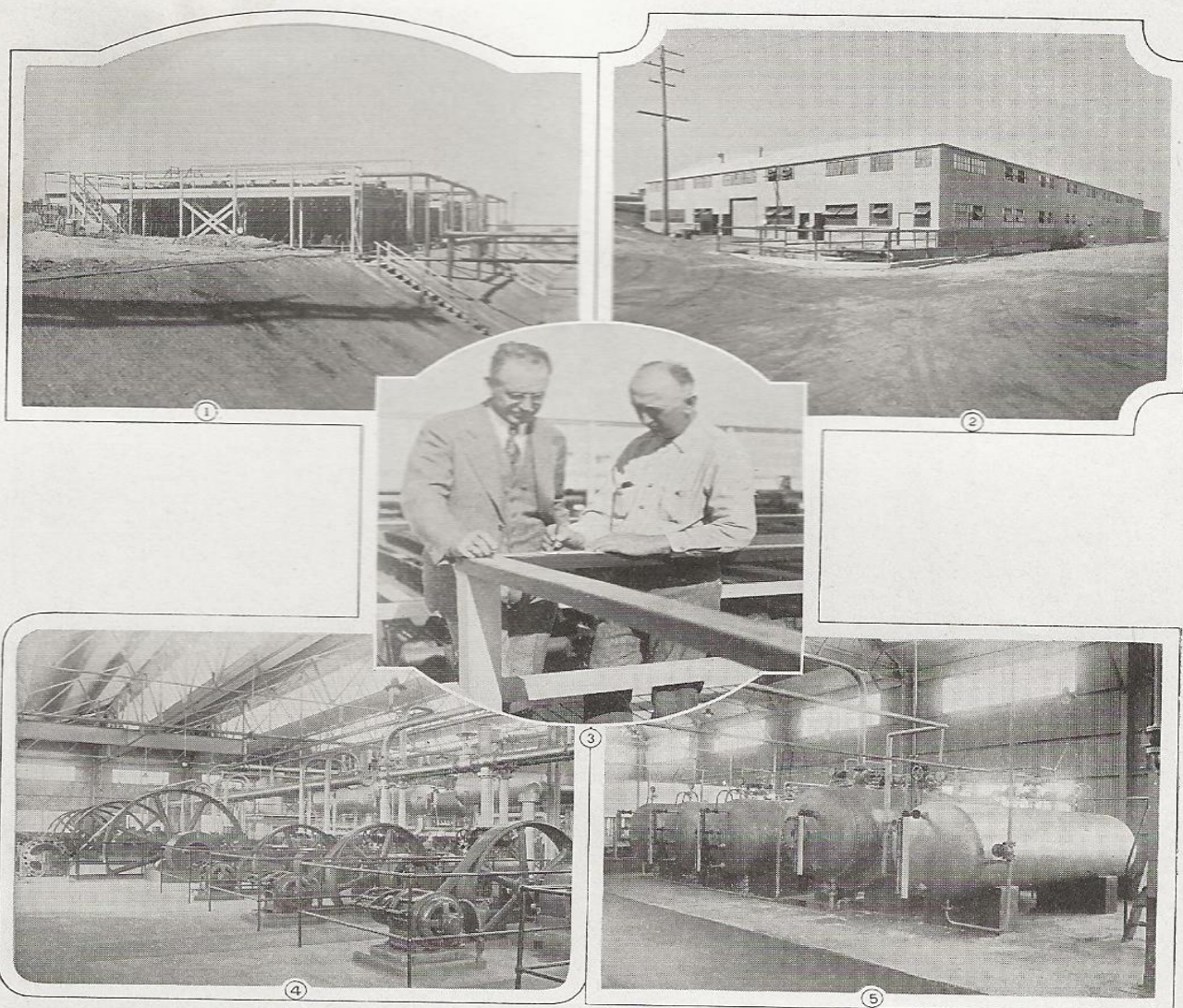
No. 1—Sulphur dioxide condensers in which the gaseous sulphur dioxide is cooled and returned to liquid state. No. 2—Exterior view of plant. No. 3—Konstantin Stolbe, (right) erecting engineer, who supervised building of plant for the German company, discussing details of condenser operation with C. M. Hoag (left) technical assistant in the Manufacturing Department in charge of electrical engineering. No. 4—Battery of vacuum pumps in foreground, and five sulphur dioxide compressor with synchronous motors in the background. No. 5—Liquid sulphur dioxide storage tanks.
