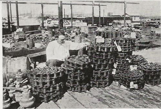
A corner of the salvage yard is devoted to castoff rotary chains. The photograph at the right shows a few of the same chains after they had been reconditioned and made ready for service.
