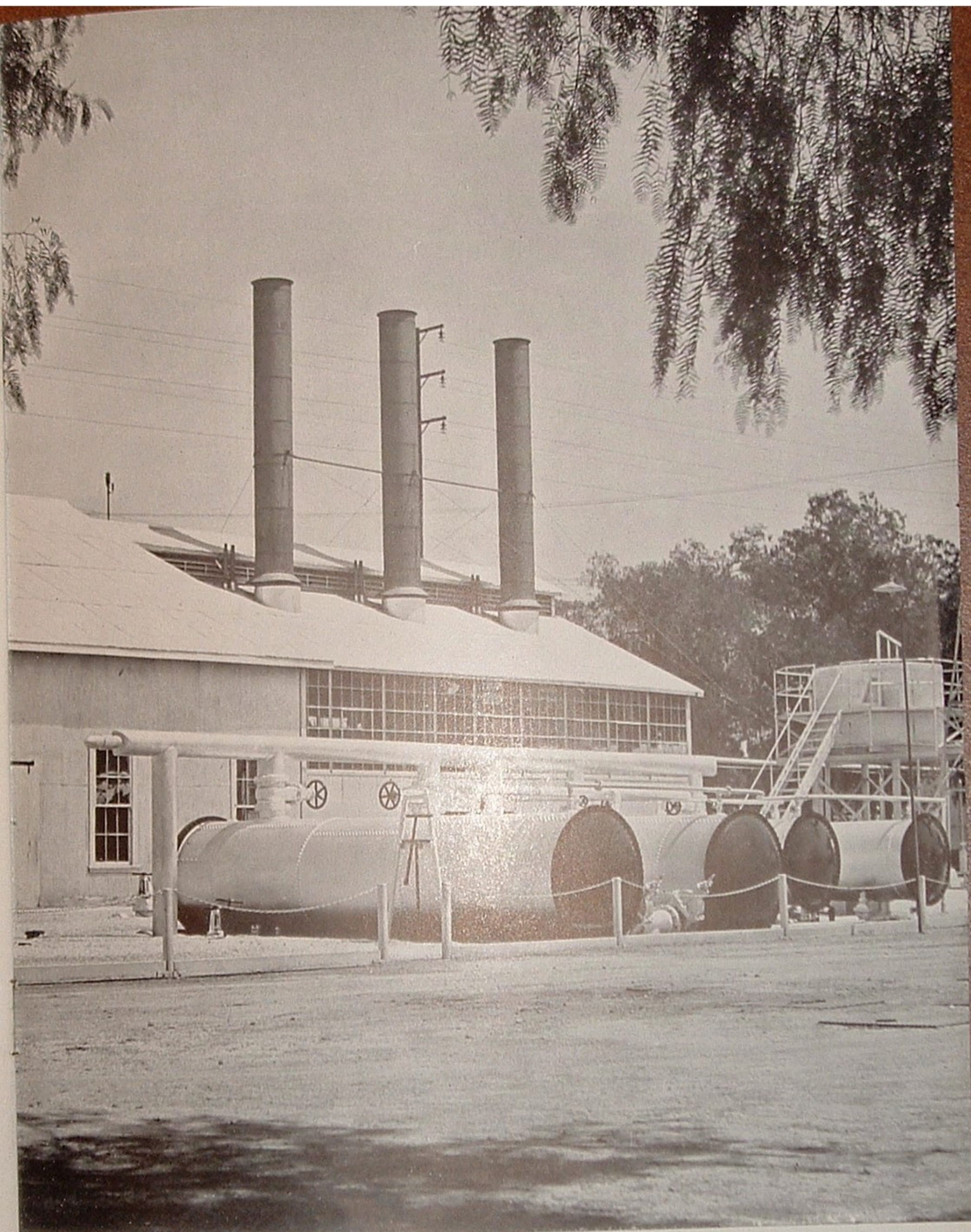
NORWALK PUMP STATION is the main power on Union's Southern Division pipeline system. Through the Southern system's 373 miles of line travel approximately 20,000,000 barrels of oil and gasoline every year, or 43,000 barrels every day.
