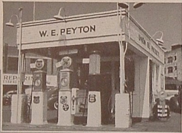
When W. E. Peyton, downtown dealer, tore out the old station at left and put in the modern unit shown below, business jumped some 30%.
