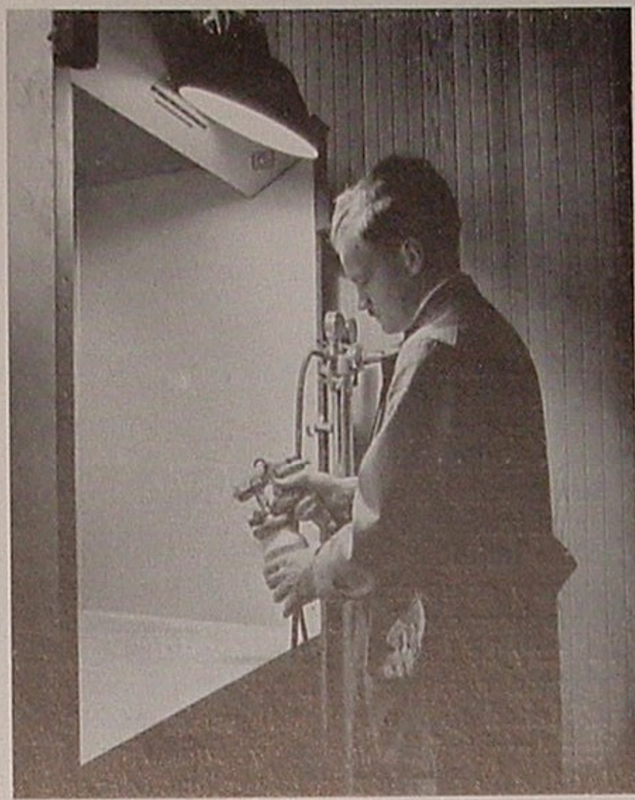
This is a spraying booth in the Pabco laboratory. Here paint is prepared for testing.
