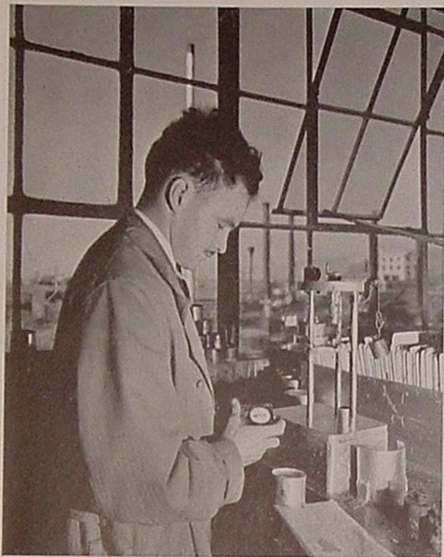
All paints and liquid ingredients are tested for viscosity in the Stormer "Viscosimeter."
