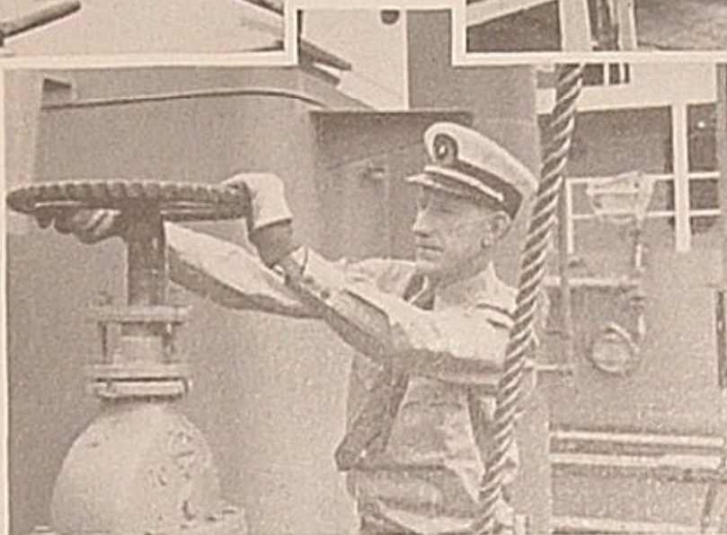
Right: Chief Officer L. L. Lishman, opens one of the gate valves into the oil tanks.
