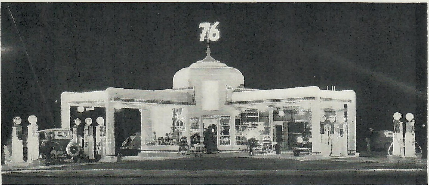
On the new civic circle at the northern entrance into Bakersfield, Calif., this modernistic, 10-pump station was opened last month by Union Service Stations. The location is one of the most strategic on the entire inland route from San Francisco bay cities to Southern California. Initial gallonage exceeded expectations.
