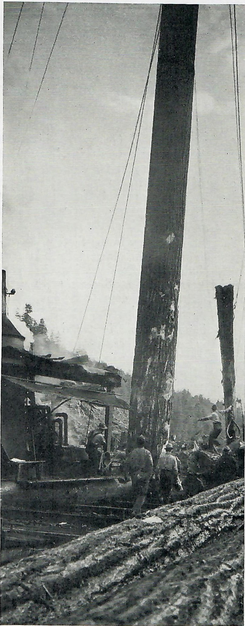
Some fast action during loading of logging train. The logs are lifted by cables run through blocks at the top of the spar tree, center, and attached to a drum on the donkey engine at the left.
