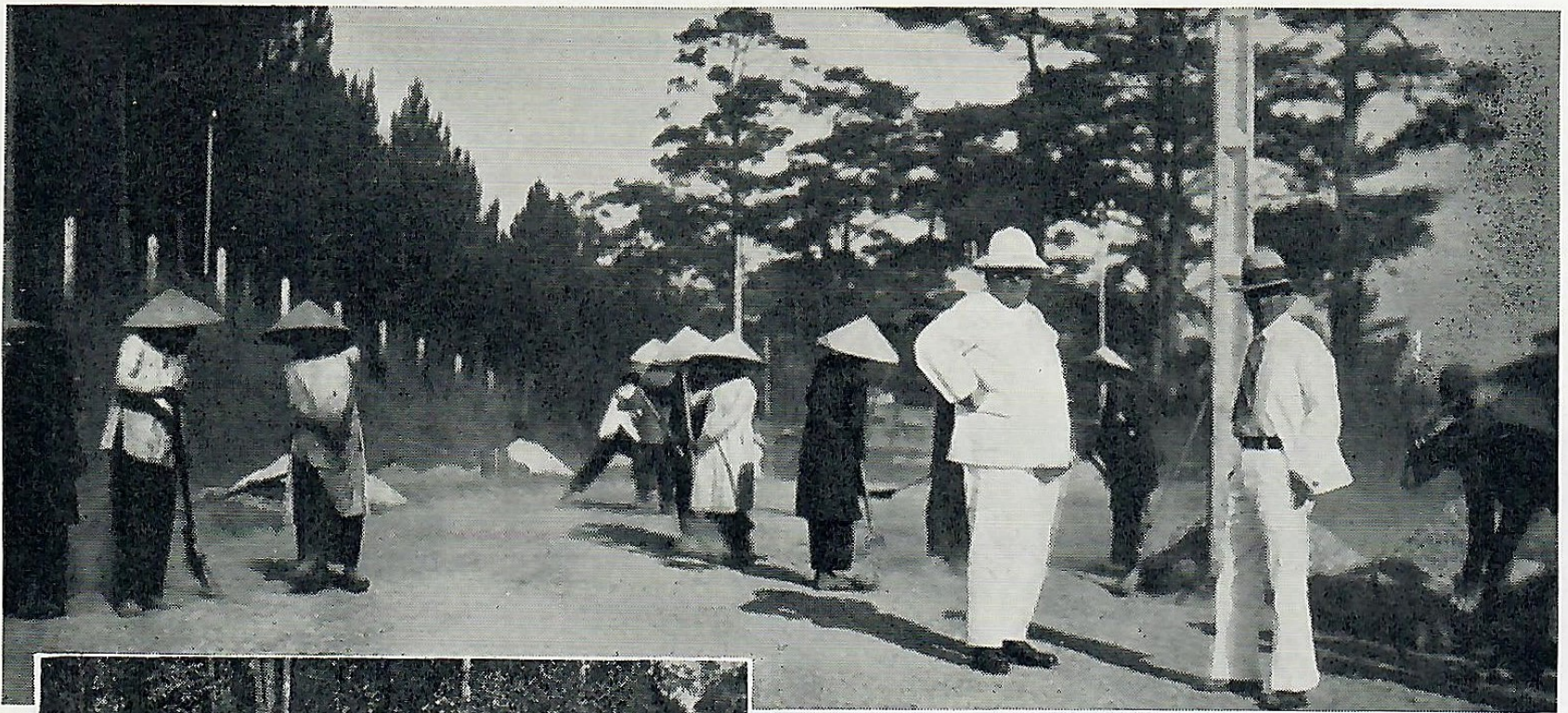
Building roads in Indo-China. The section of highway shown above is to be surfaced with Union emulsified asphalt, heavy. The work is being done by native women. A. Guyonett, Union's lubricating oil agent at Saigon, is shown in center. At the left native labor is preparing roadbed through jungle. Union asphalt will be used on this job.
