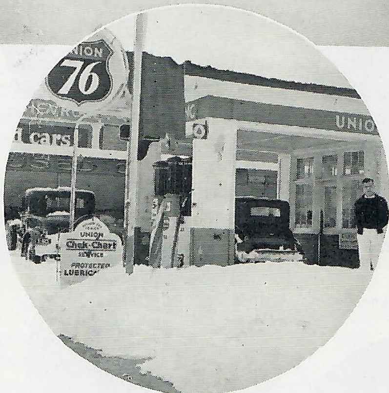
Reno substation and Union Service Stations, Inc., No. 37, Virginia and Court streets, as they looked following storm of January 21 when 16 inches of snow fell.
