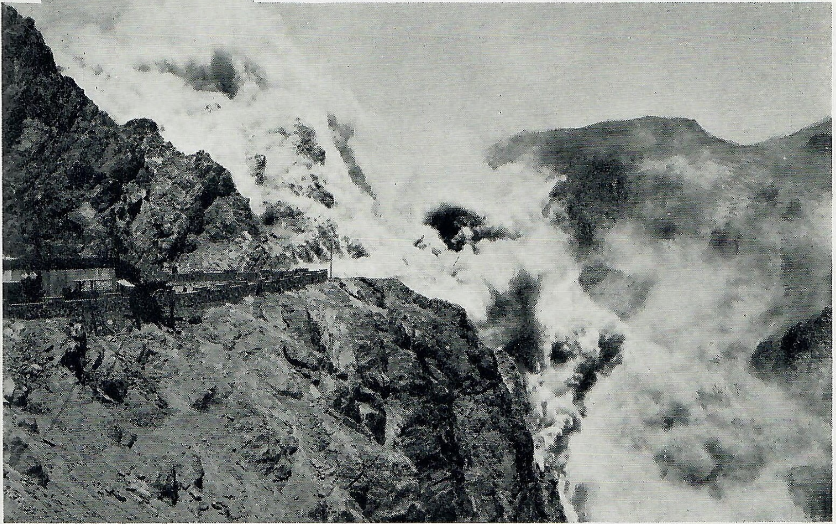
Dynamite speeds work at Hoover Dam
