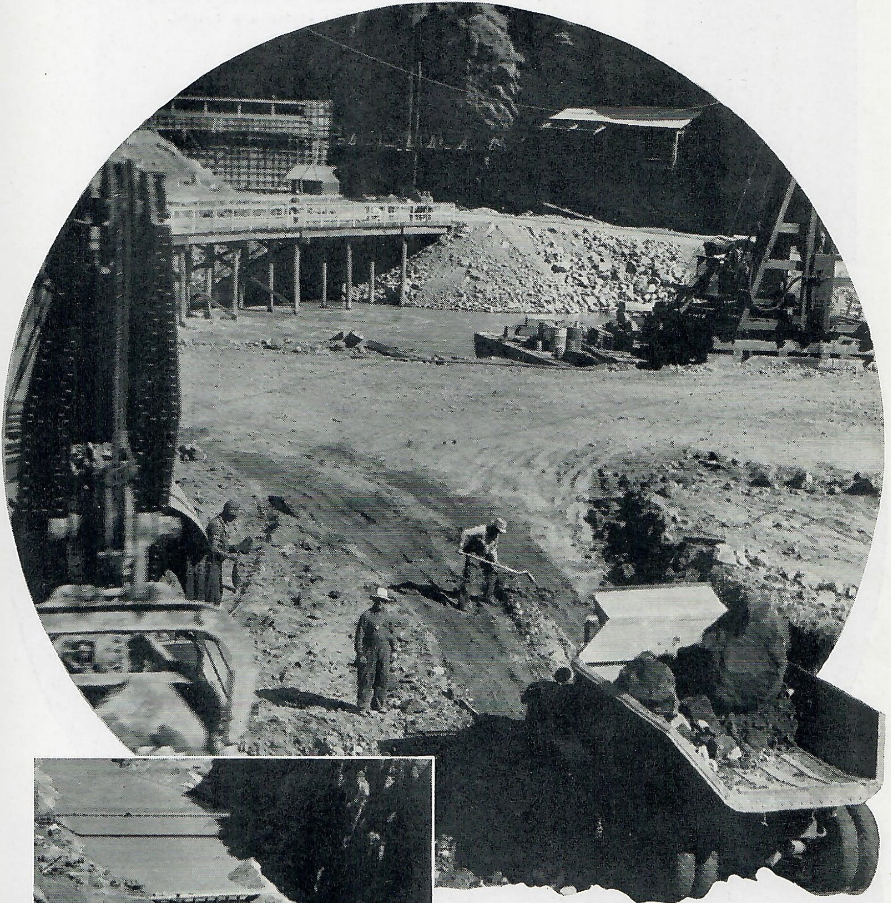
Construction of the 75-foot cofferdam that will turn the Colorado River from its age-old course and into the four diversion tunnels was started Sept. 20. The photograph in the circle shows work in progress on the coffer dam, while the lower picture shows the rock fill that has been extended part way across the river preparatory to building the dam.
