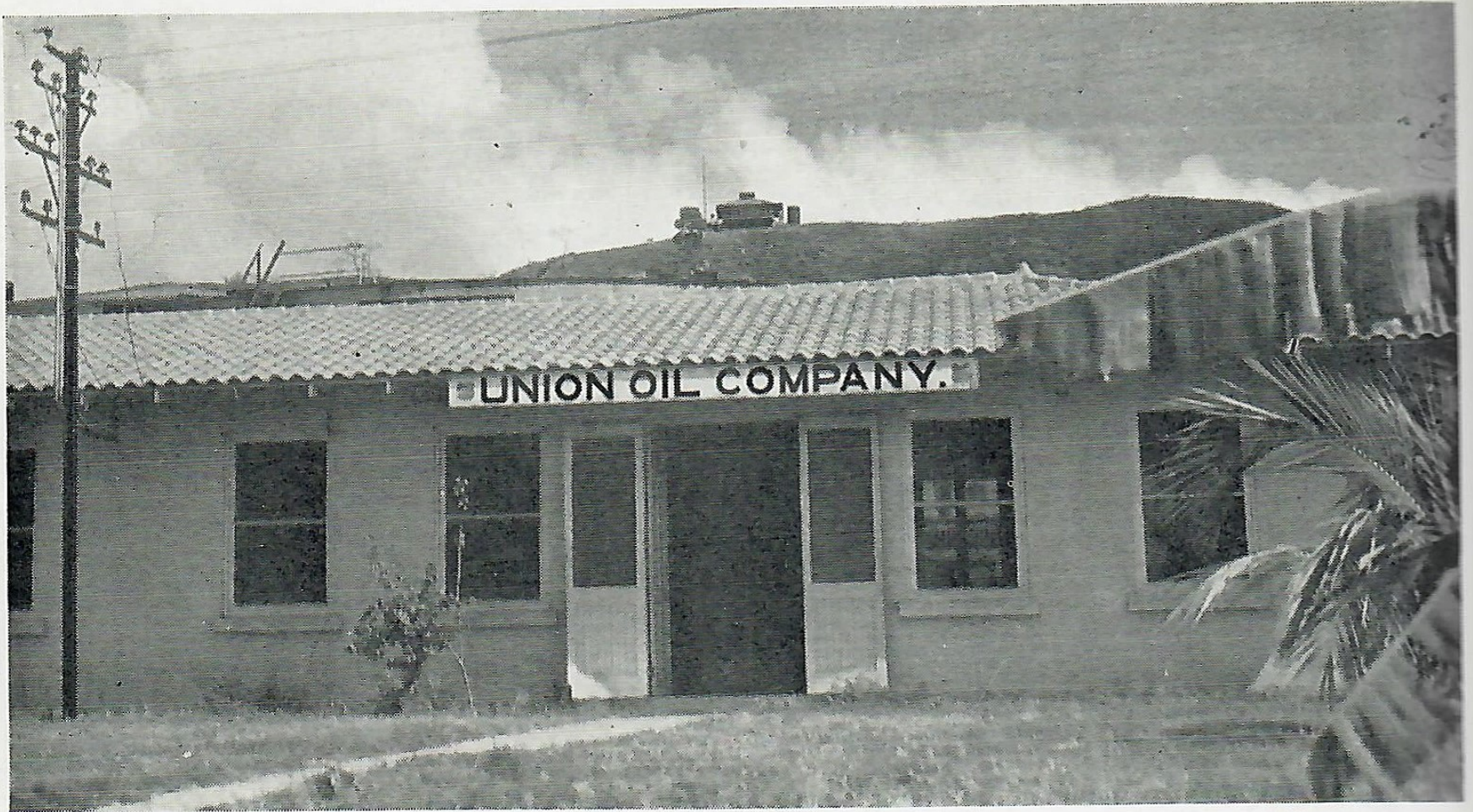
Company's headquarters for Panama, Union Oil Place, Balboa, Canal Zone.
