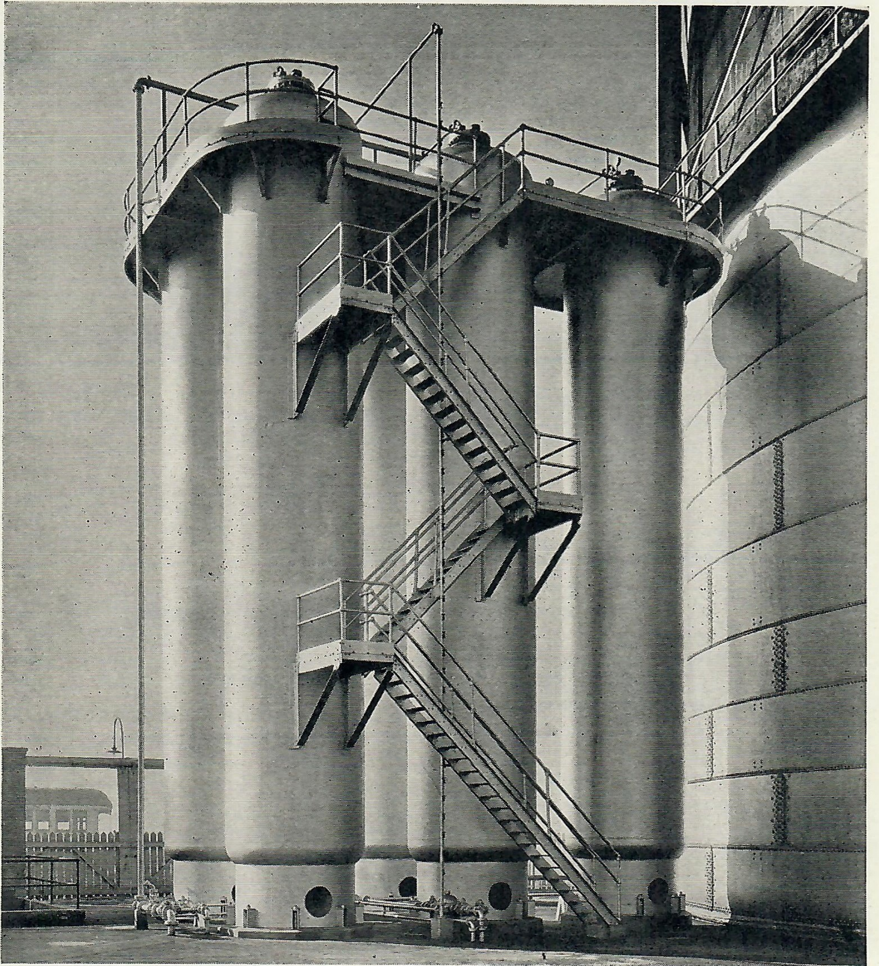
The five liquid gas storage tanks supplementing oil gas manufacturing equipment at San Diego Consolidated Gas and Electric company's plant have combined capacity of 75,000 gallons. The vertical pipe running up through stairway is novel gauging device by means of which amount of liquid gas in any one of the five tanks can be immediately determined.
