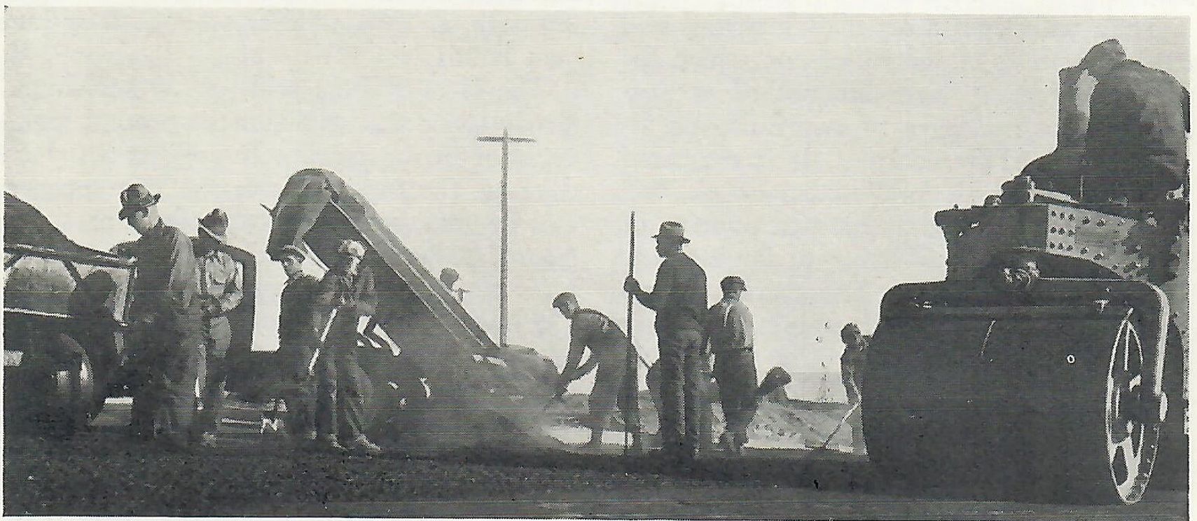
Asphalt is being used to pave the streets of Boulder City and the highways to the dam.
