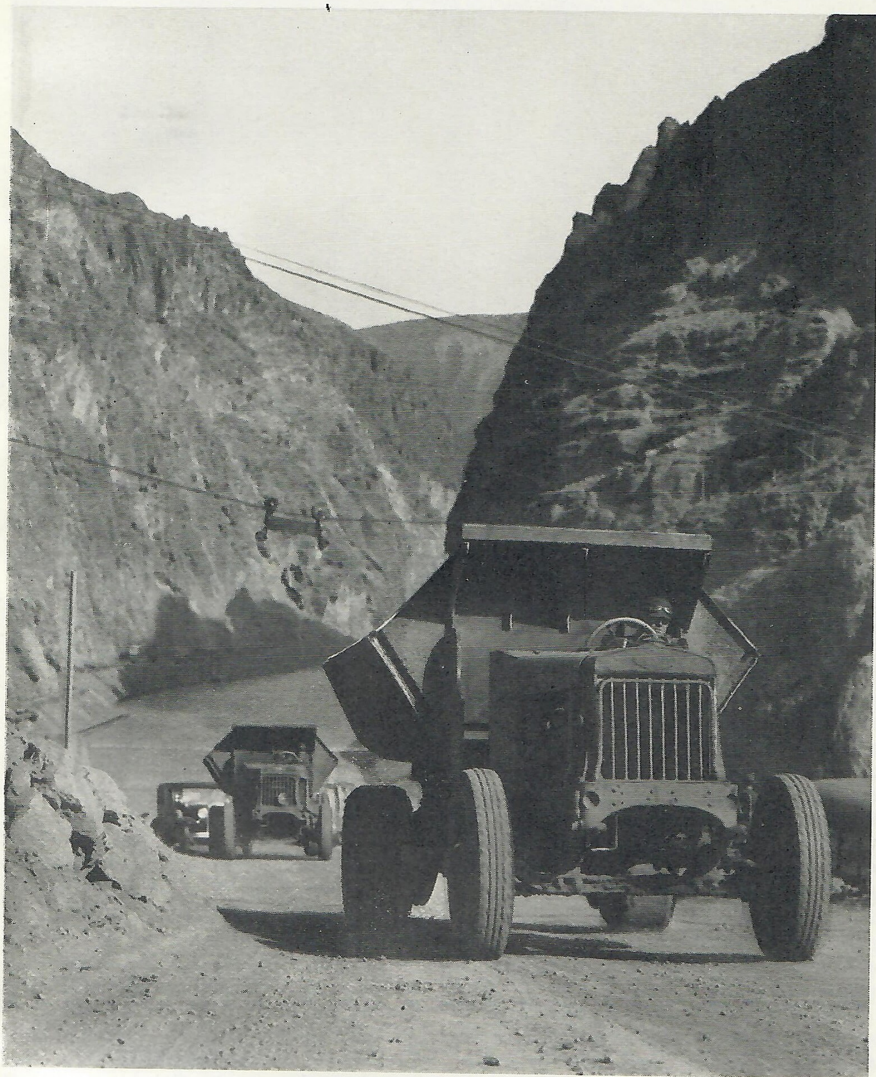
These mammoth trucks, each carrying 10 tons of rock from the diversion tunnels, are climbing the steep grade from the lower portal of the dam. The trucks are driven into the tunnels, which are 56 feet in diameter, and are loaded by steam shovels.
