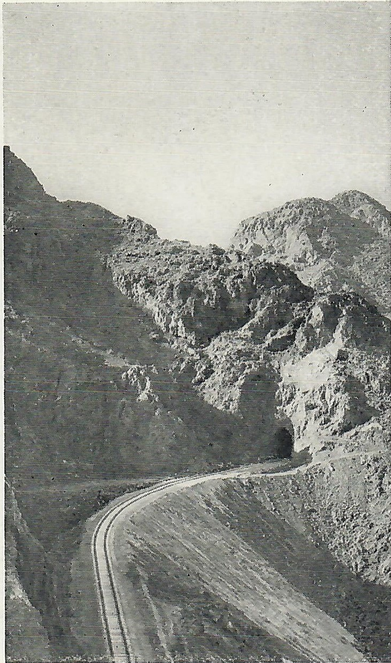
The building of the Hoover Dam railroad, a section of the right-of-way of which is shown above, is one of the outstanding feats of the entire project. Virtually every foot of the way of this short rail line, which penetrates volcanic rock peaks and skirts along the perpendicular walls of Black Canyon to the water's edge, had to be blasted.
