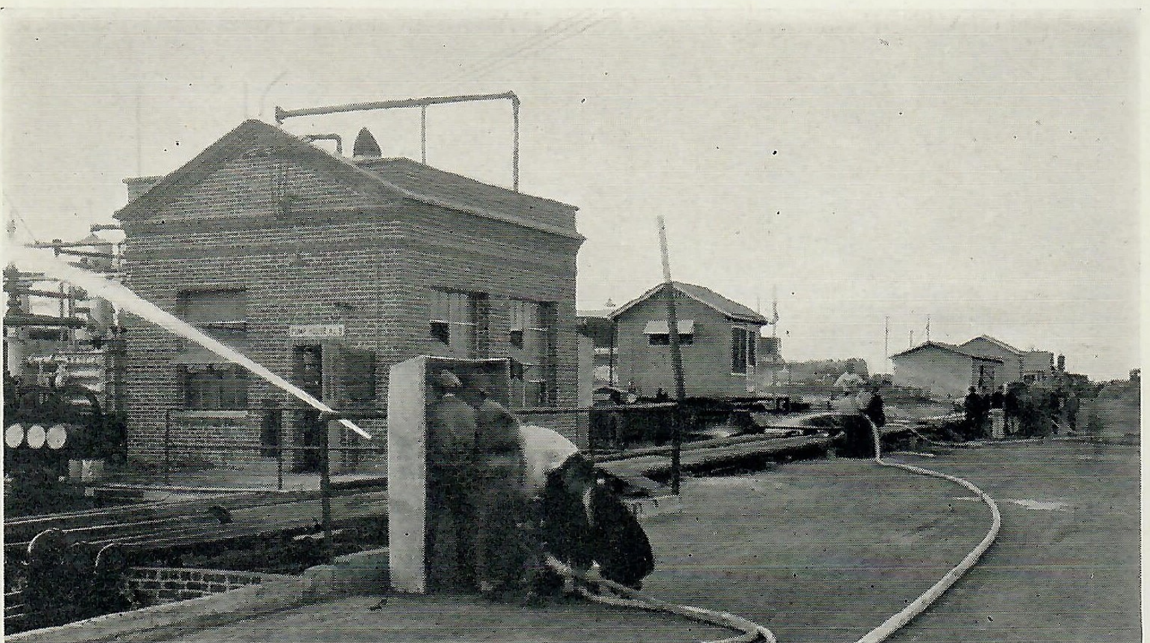
Typical hose drill. This is made part of the training of all refinery shift men.
