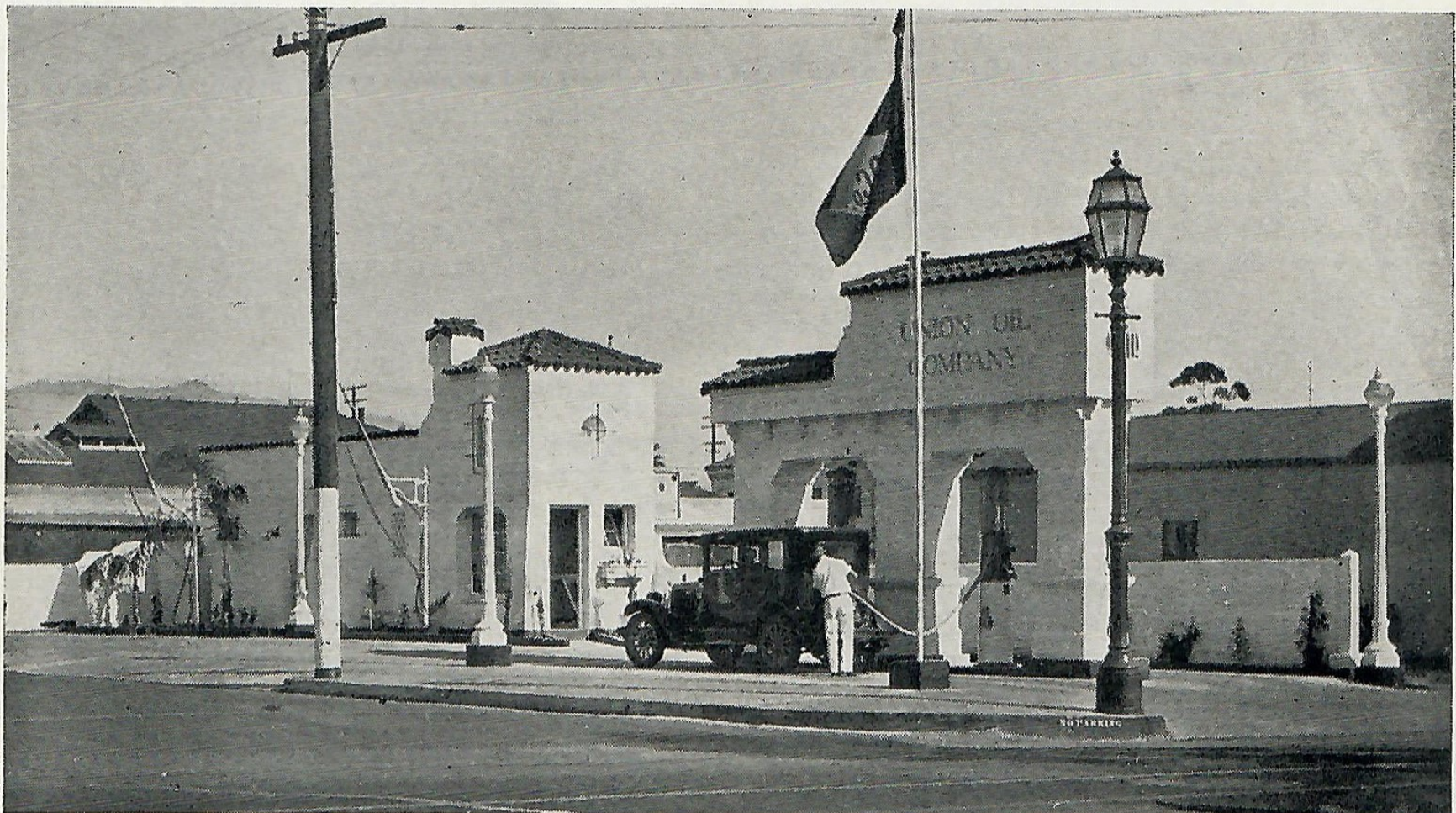
Union Oil engineers put model service station on 30-foot lot in Santa Barbara.
