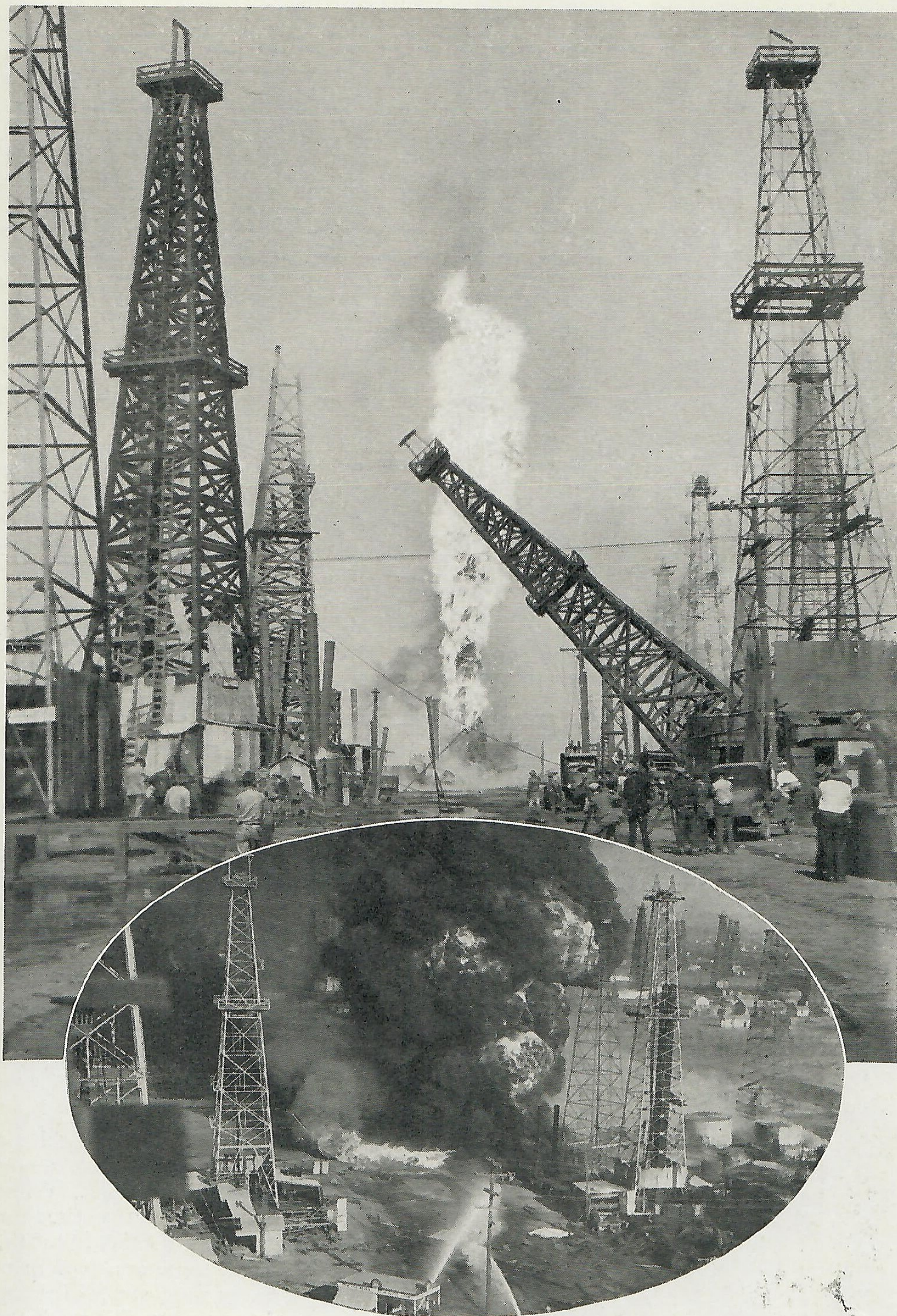
The remarkable photograph at the top of the blazing Bellview Syndicate well at Santa Fe Springs was snapped by Fred Coffey, Times' staff photographer, just as one of the wooden derricks, being wrecked to prevent the spread of the fire, toppled over. The lower photograph is an impressive picture of the Getty No. 17 which burned for fifty days.
