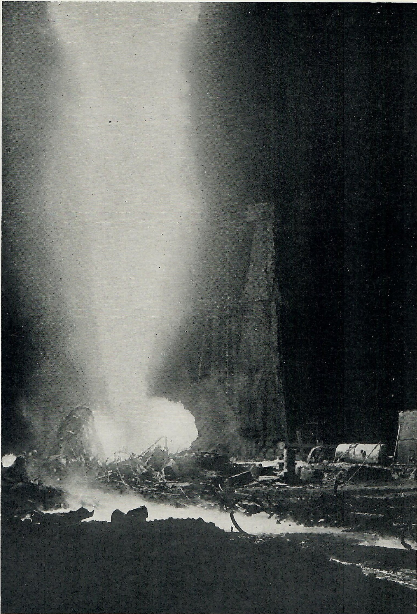
Asbestos-clad workmen in "Dante's Inferno." This dramatic photograph taken of the Bellview well at night by A. R. Hromatka shows how the fire fighters braved the intense heat to remove the debris blocking the way to the well. The scrap heap in the foreground shows difficulties which confronted workmen. This photograph cost the cameraman a lens.
