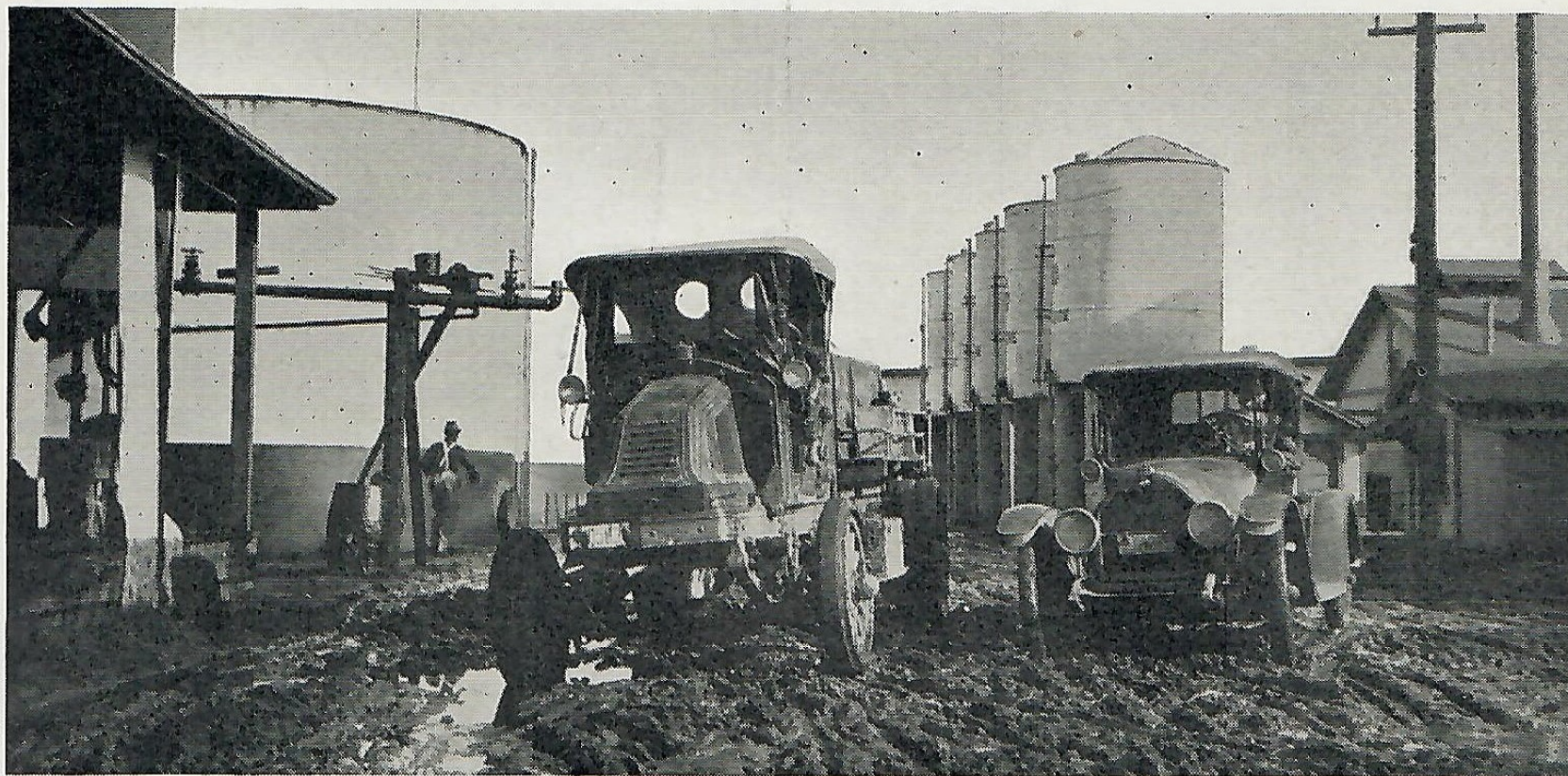
Winter scene at main San Diego distributing plant in 1915.
