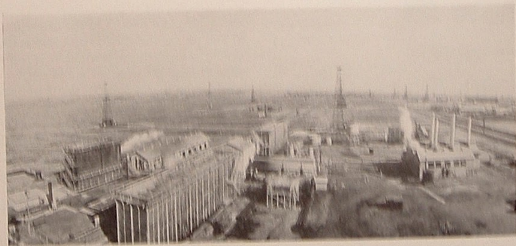
General view of the Dominguez Absorption and Compressor Plants
