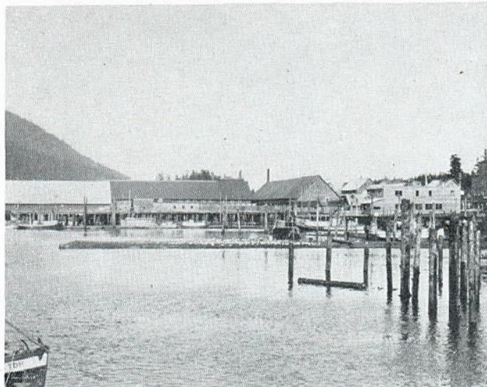
Portion of the harbor at Petersburg, our most northern Alaskan station. Note how all the buildings are placed on piling above the water.
