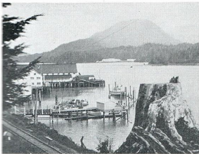
Inverness, B. C., showing cannery, warehouse and Union Oil dock. Here the water is 1½ feet deep at low tide and 22 feet deep at high tide.
