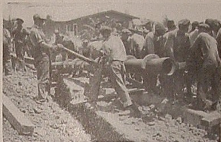
CONSTRUCTING A PIPE-LINE
