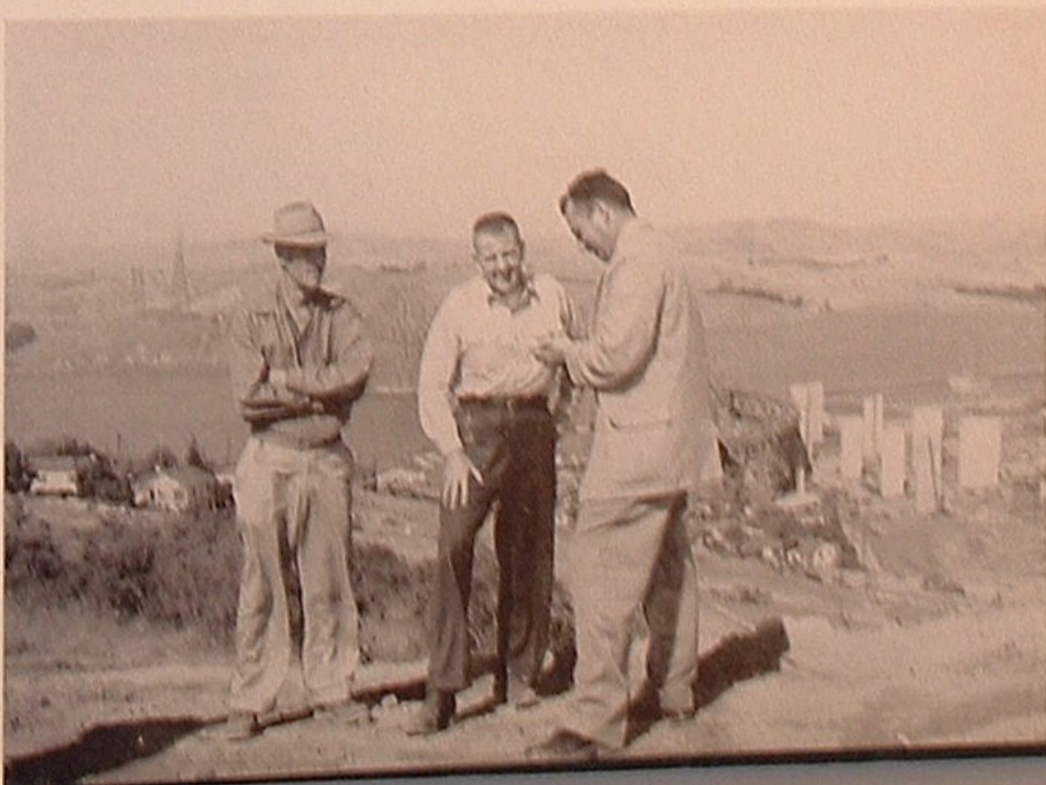
From left, California Division of Highways Engineers H. C. Tunks, C. P. Sweet and V. O. Smith discuss progress of the job near Crockett. Concrete structures, extreme right, will support the new bridge across Carquinez Strait.
