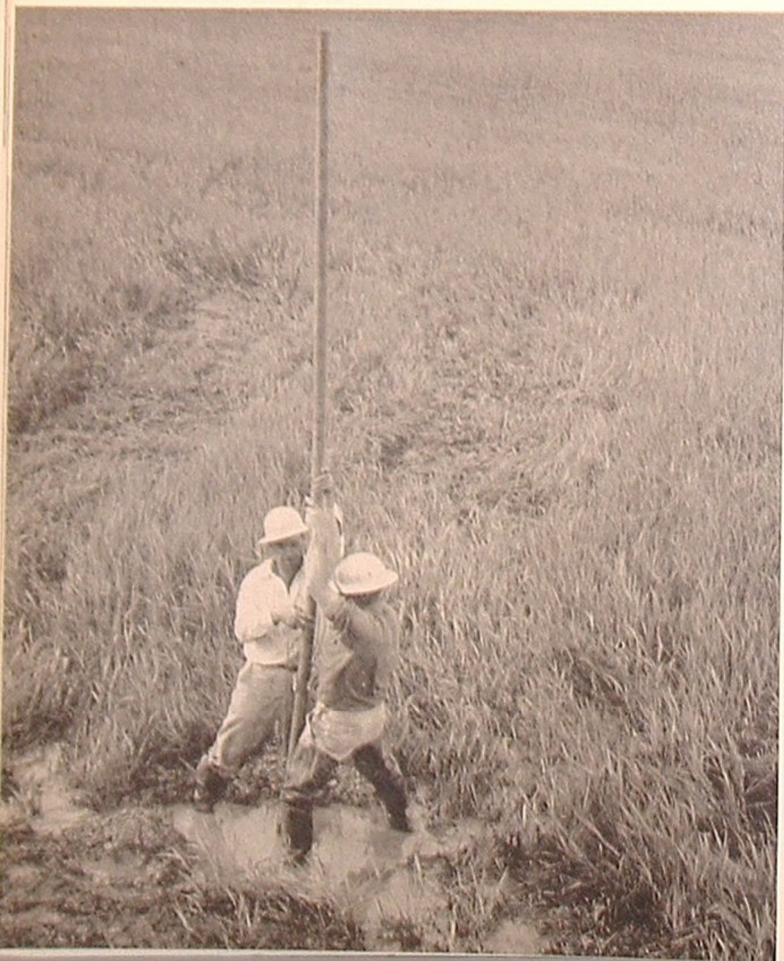
At left, two Cajuns are ramming an explosive charge into one of the shot holes. Below, a cable-jug-boat, towed by marsh buggy, pays out several hundred yards of insulated cable equipped at 120-foot intervals with geophones (jugs). When the charge is exploded, jugs will change earth vibrations to electrical pulses.
