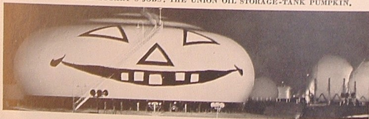
ONE OF DARRELL STUART'S JOBS: THE UNION OIL STORAGE-TANK PUMPKIN.
