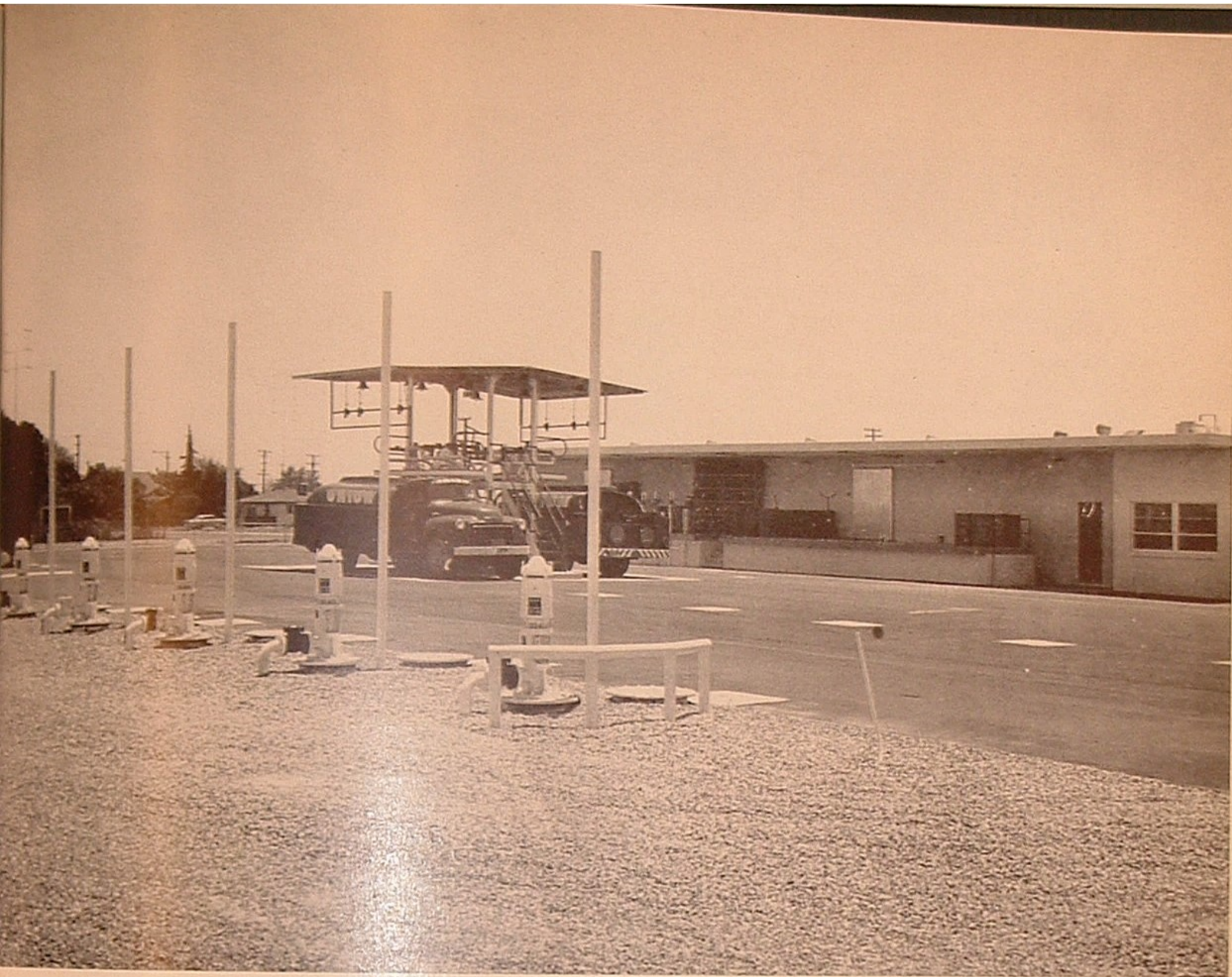
Made conspicuous by their disappearance are the conventional above-ground storage tanks. At Bakersfield, five 20,000-gallon tanks are buried underground. Only vent pipes and electric motors hint as to their whereabouts. Valuable property above the tanks now has other uses.
