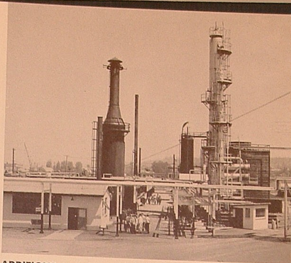
ADDITIONS recently made to our Edmonds Refinery near Seattle now enable the Company to manufacture several airblown asphalts in addition to the paving asphalts made here. The photo was taken during a May inspection by employees of both the refinery and its terminal.
