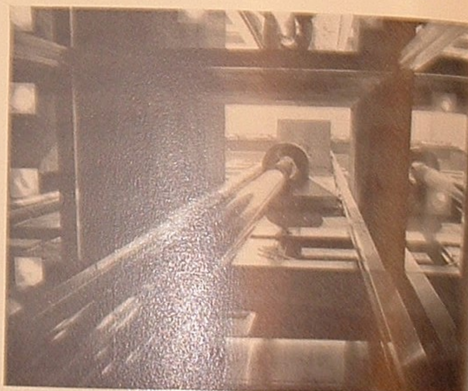
Above are two views of the 162-foot ram, whose 25,000-pound load is supported on a column of oil. The collar halfway up the shaft is a follower-guide used to guard against swaying of the ram during high winds. Below, Union Oilers Vic Morrison and Walt Bassett of San Diego hear a technical description of the elevator by Dick McIntyre and Arnold Hunsberger, two of its three builders.
