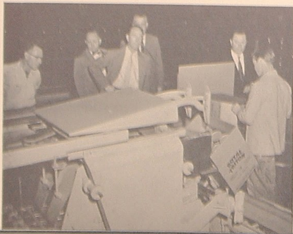
At right, Ira Shearhart demonstrates the fast machine-filling of Royal Triton cartons, 24 cans to the case.
