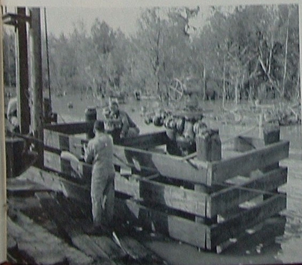
Below, workmen are building the platform for another development well. At right are Division Superintendent Ed
