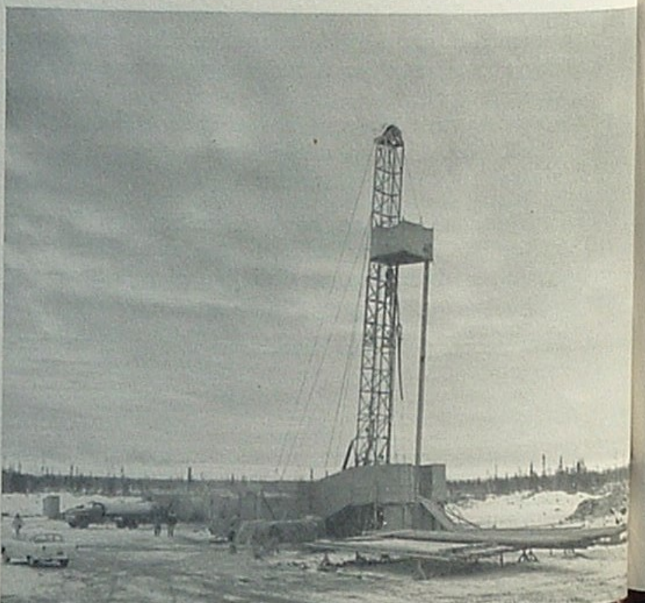
"Circulation has been restored at Loon River, below. 'The party smiles. Over hot coffee (above) Grinsfelder, Kerkhoff and Bob Roethke decide to seal off the porous zone with casing and postpone completion till December.'"
