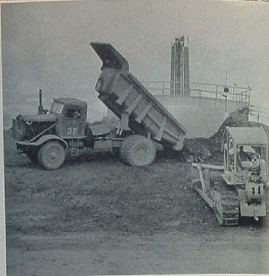
After being shovel-loaded, the 22-ton Euclid dump trucks start the ore through a crushing and screening plant.
