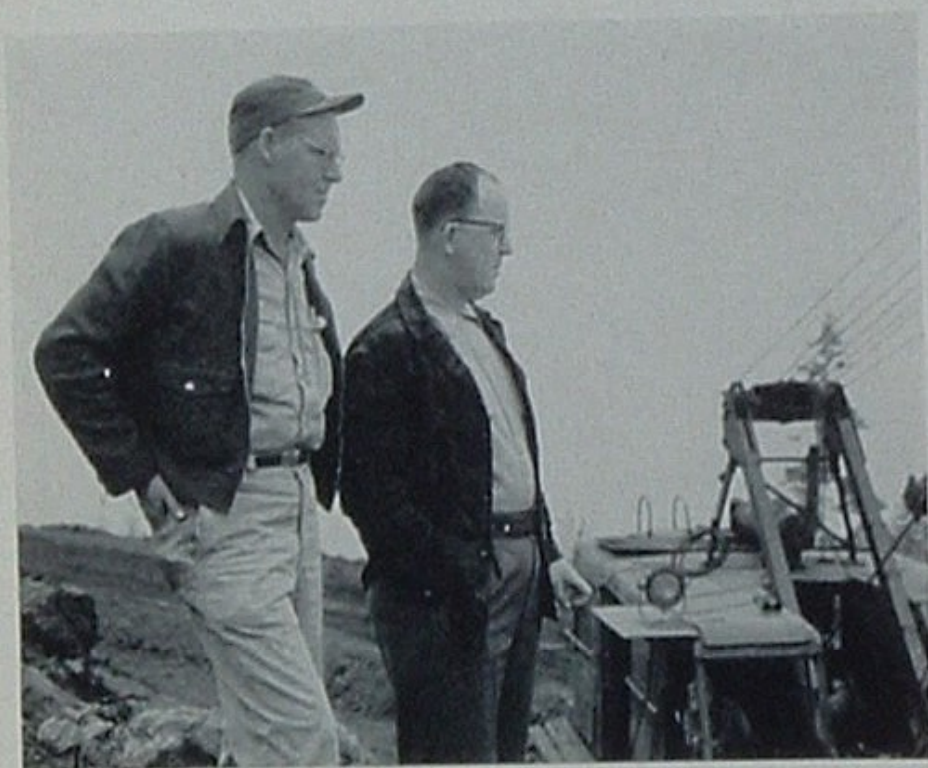
Above are Mine Foreman Henry Servant and Consignee Don W. Clark, who keeps the project supplied with Union Oil products. At right, an 8,300-foot tramway carries the ore downhill to the Hanna smelter, meanwhile generating sufficient electricity to satisfy local power and light needs.
