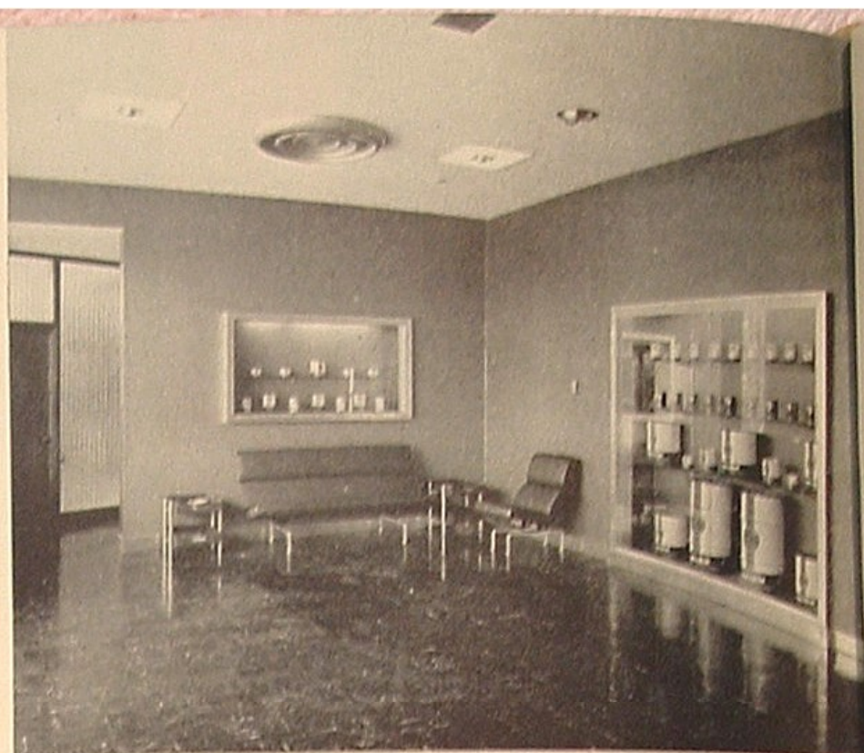
Union Oil Building's new entrance lobby
