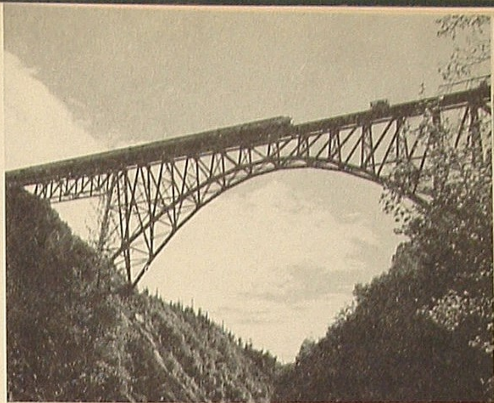
Some 235 miles inland from Whittier, Union Oil tank cars cross Hurricane Gulch via this bridge—to Fairbanks.
