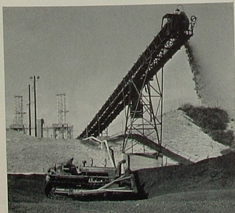
Above, the control room from which both coking units are operated represents the most advanced instrumentation. Below, byproduct coke drops from the end of a long transfer conveyor for storage pending its eventual use in the manufacture of electrodes, lamp black, and so on.
