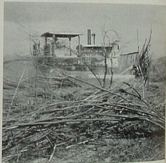
Tractor driven rakes push the uprooted brush into piles or windrows, above. Later the debris is sprayed with oil and carried away by one of man's oldest servants—fire, below.
