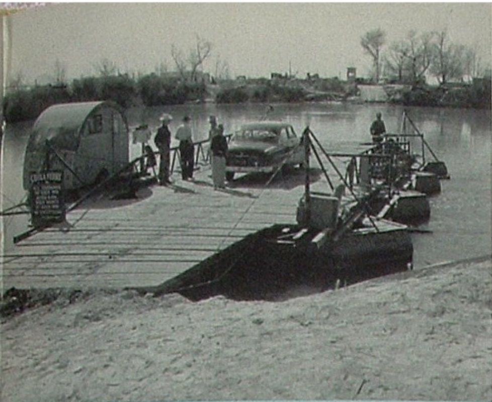
This current-powered ferry takes men and equipment to clearing operations on both sides of the Colorado River. Its profits also keep the access road open to Blythe.
