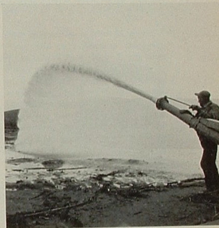
Below, at Fairbanks water is used to wash away 100-ft. overburden of muck.
