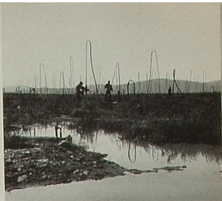
Arctic ground, frozen to bedrock, must be thawed before dredging begins.
