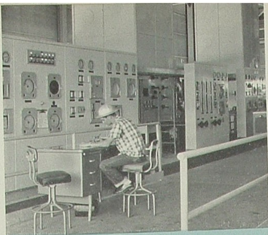
INSTRUMENT PANEL —Scrubbing of the crude hydrogen gas stream is observed and regulated at this gas-reforming control board by Operator Donald Fox.
