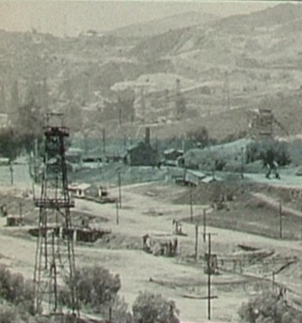
NATURAL GAS from Union Oil's Stearns Absorption Plant near Brea provides the hydrocarbons from which the remaining hydrogen requirements are obtained.
