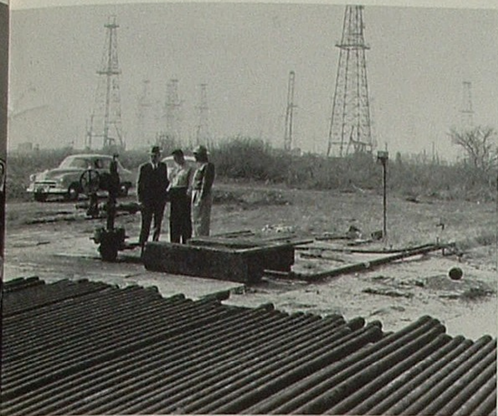
This well on the edge of our Dominguez Field carries salt water down to the oil-producing formation, creating a water flood in the direction of producing wells beyond.
