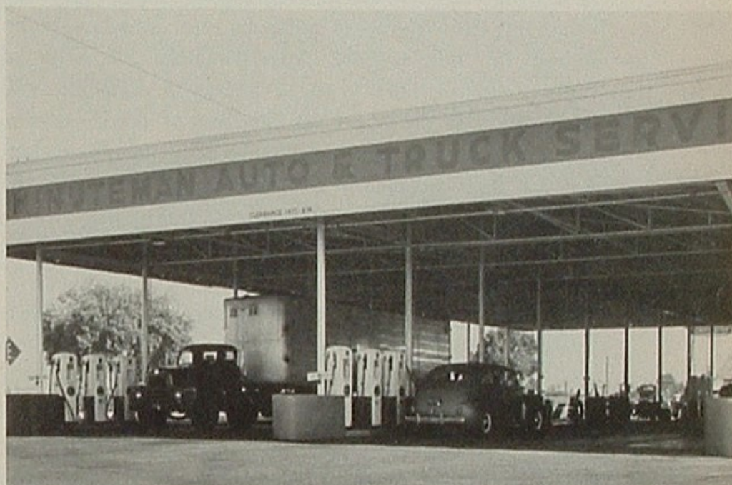
Typical of many Union Oil service units in the Fresno metropolitan area are the spacious dealer-operated truck terminal, above, and new service station, below.
