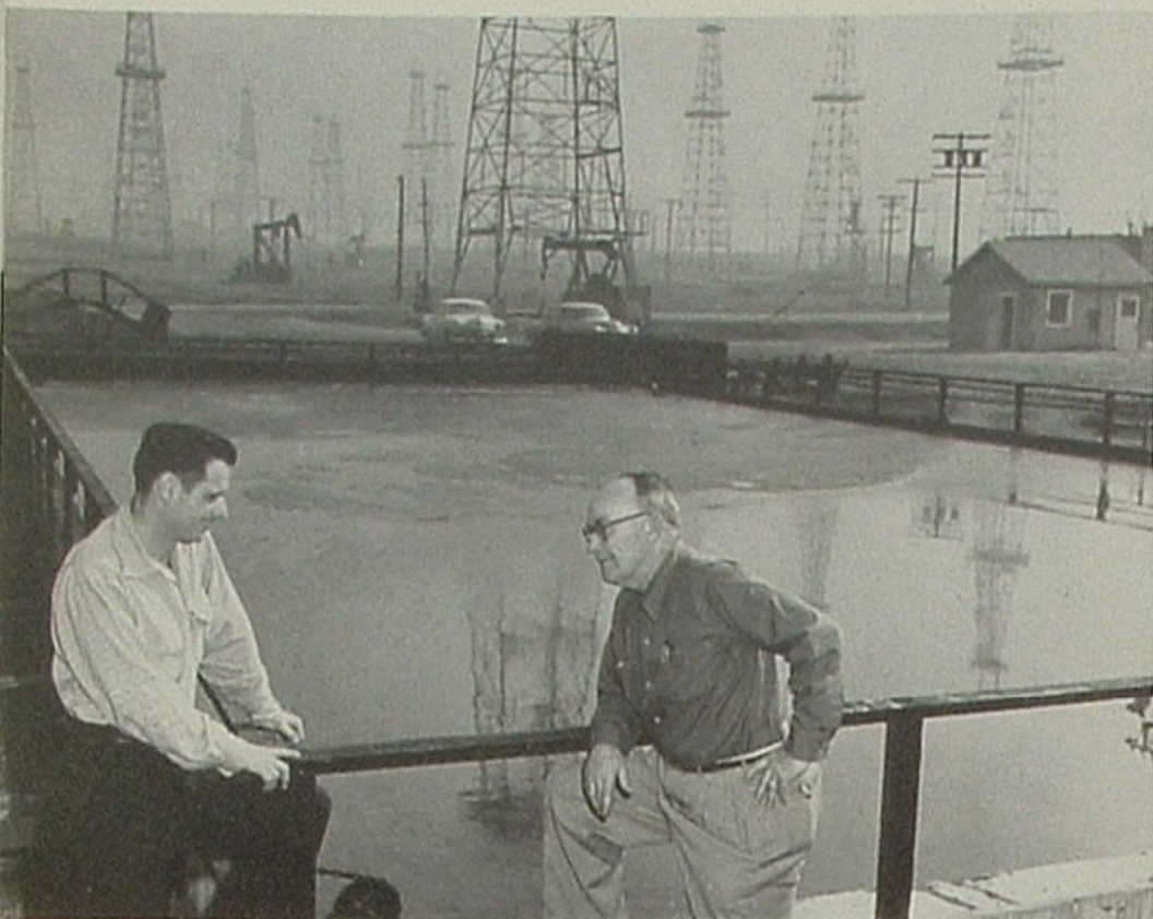
Assistant Foreman Harry Keegan and Foreman Otto Gillingham are in charge of water-flooding project at Dominguez. The briny waste in skim pond will be injected underground.
