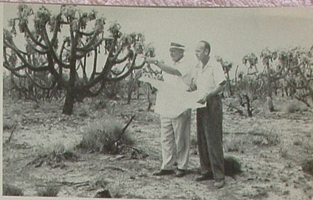
"The 76 sign goes right where that horned toad is sitting," explained Webb Construction Company's R. G. Fleming to J. E. Stephens on site of new Union Oil service station.
