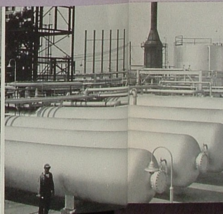
Separation of inferior from superior lubricating hydrocarbons takes place in the large horizontal tanks through
