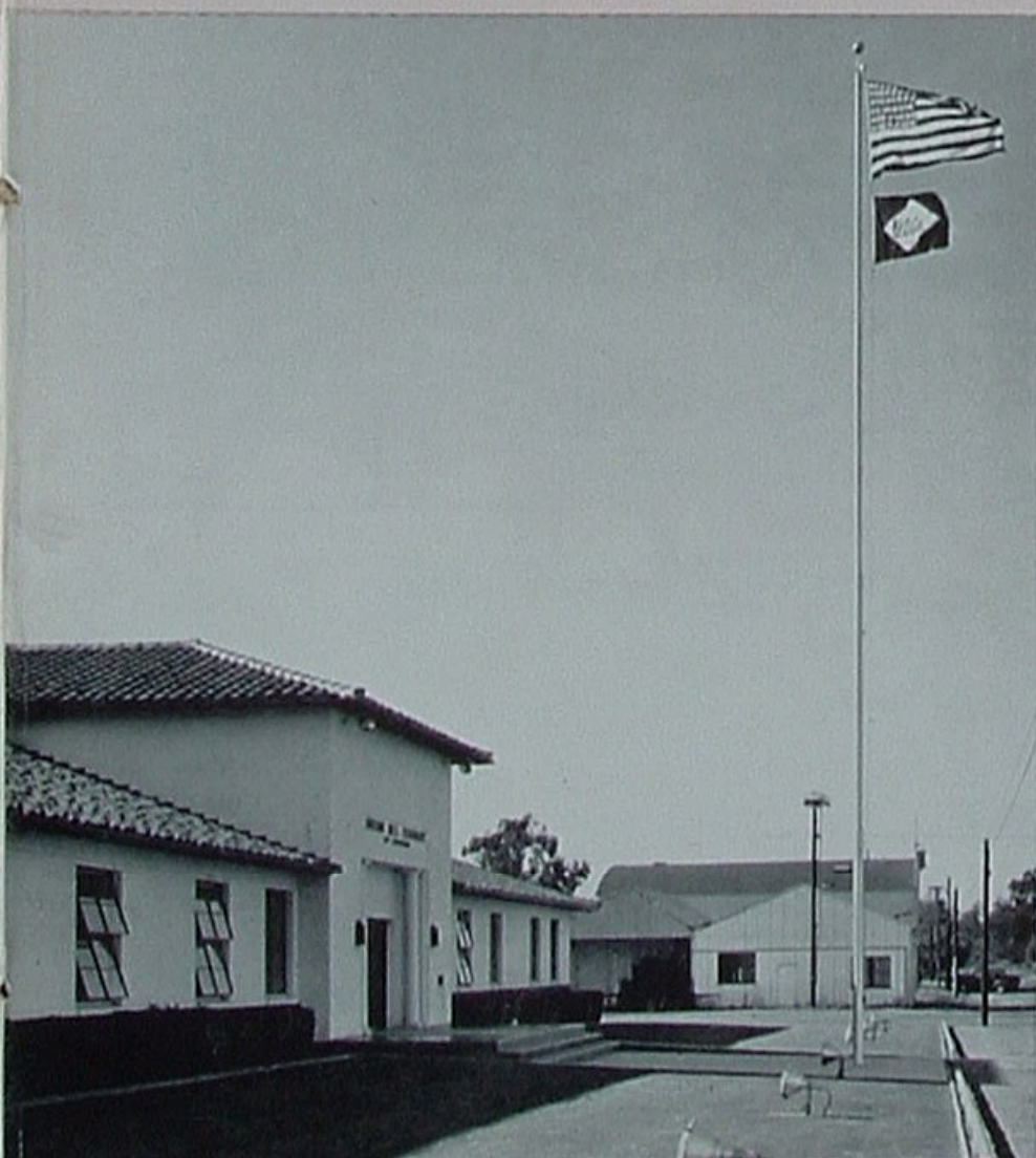
Coast Division office at Orcutt, California.
