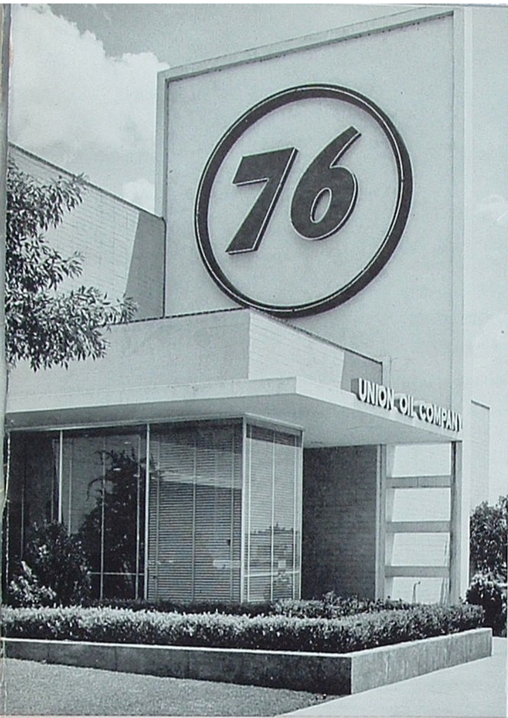
Office entrance at Bakersfield, California.
