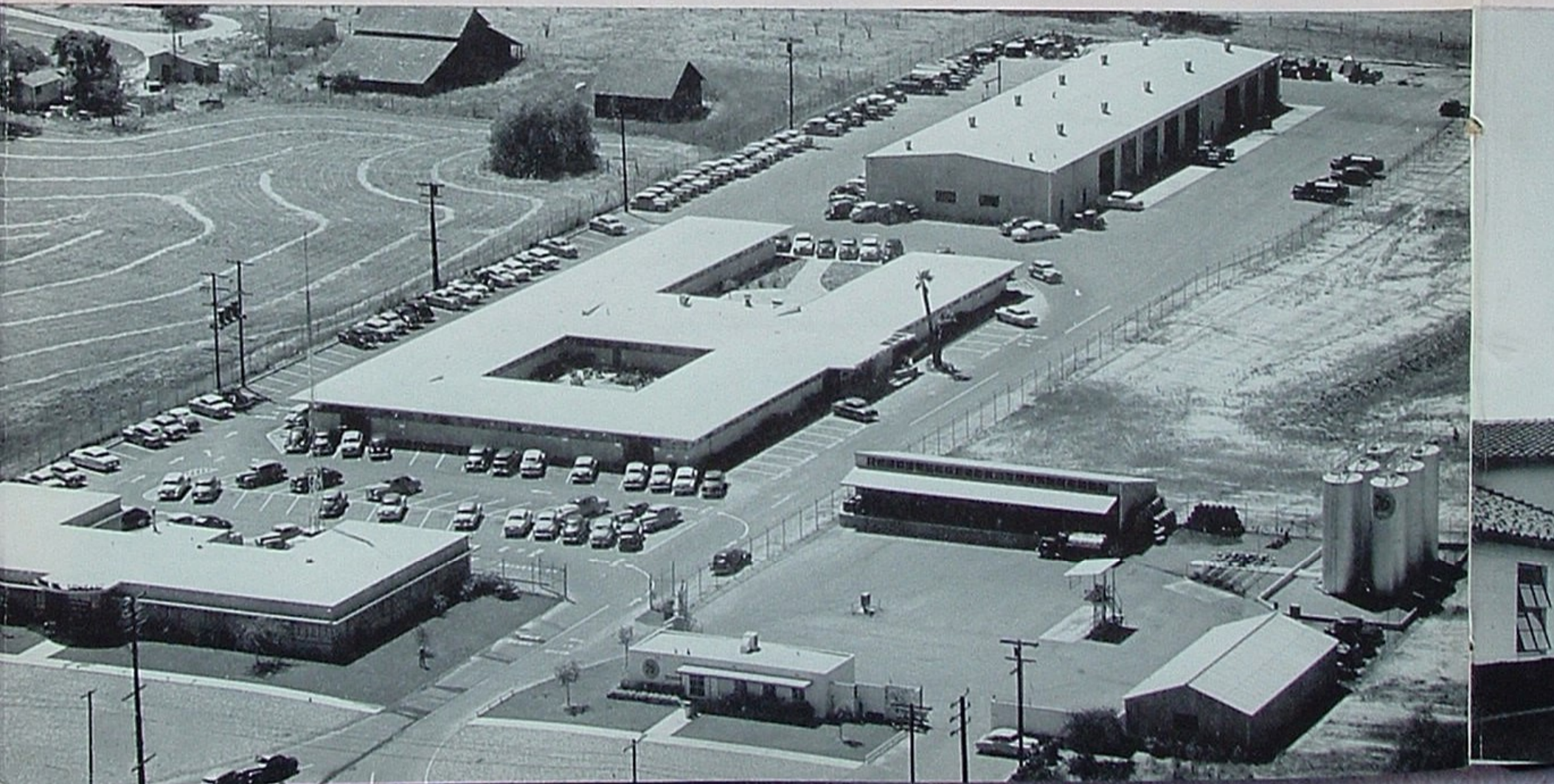
Offices and garage at Santa Fe Springs, California.
