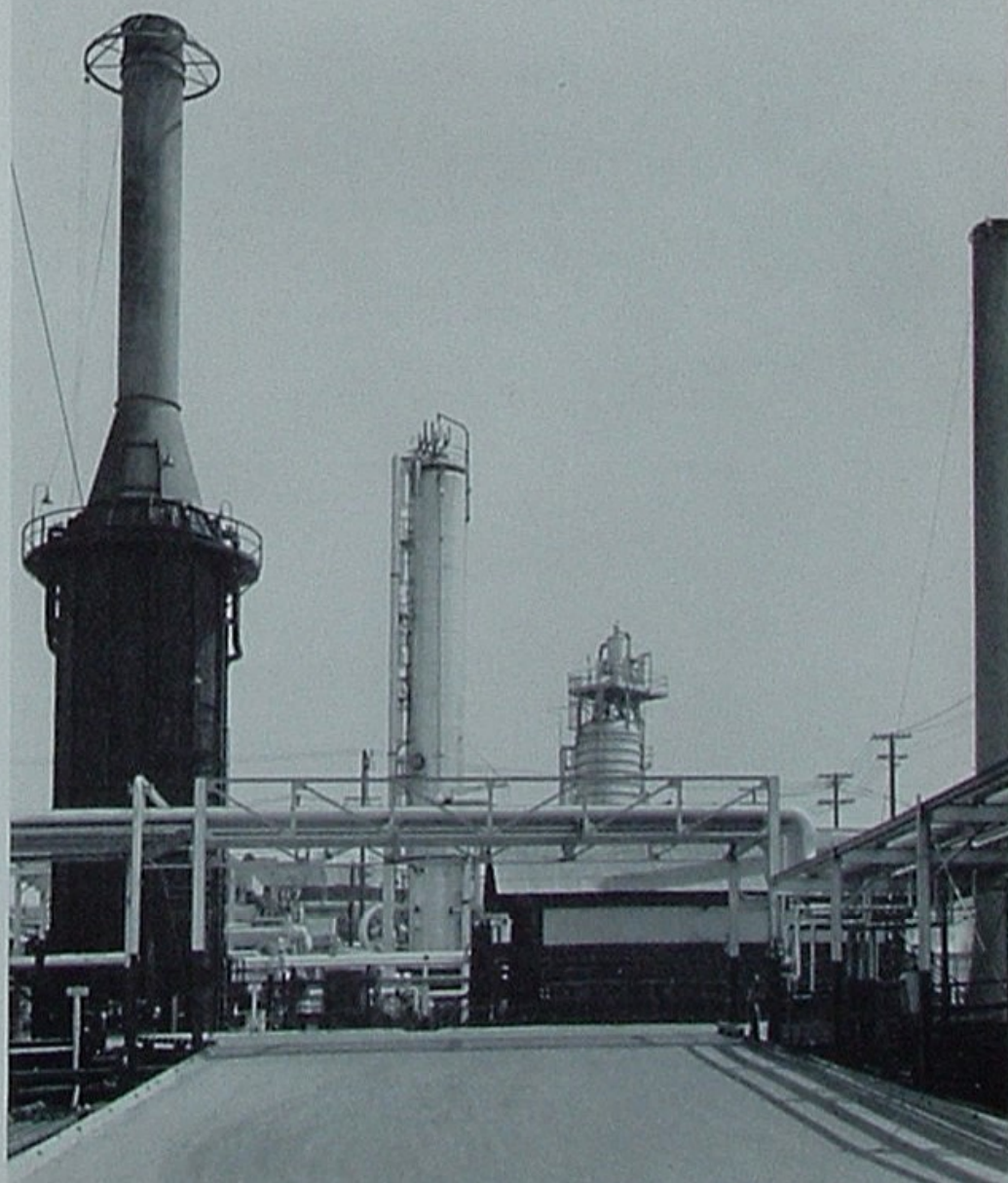
Oleum Refinery on San Francisco Bay, left, manufactures our entire output of lubricants. Heaters and columns of Distillation Unit 67, above and below, first remove light fractions from waxy crude stocks.
