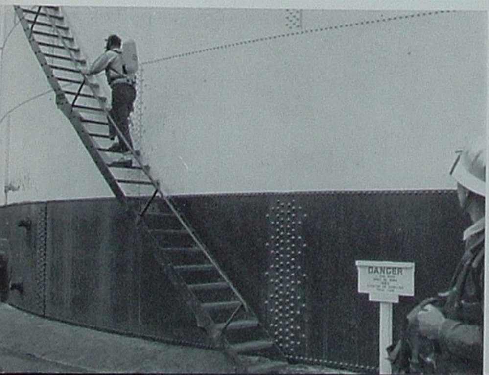
Below, a sign warns of the presence of hydrogen sulfide in this storage tank. So, the gauger breathes by means of a Scott Air-Pak and is checked by a standby observer.
