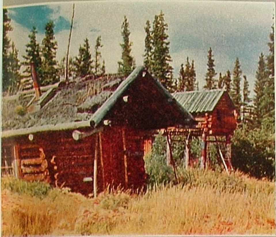
Above, 114 miles from Tok, Alaska, this sod-roofed log cabin and stilted food cache are still in daily use.
