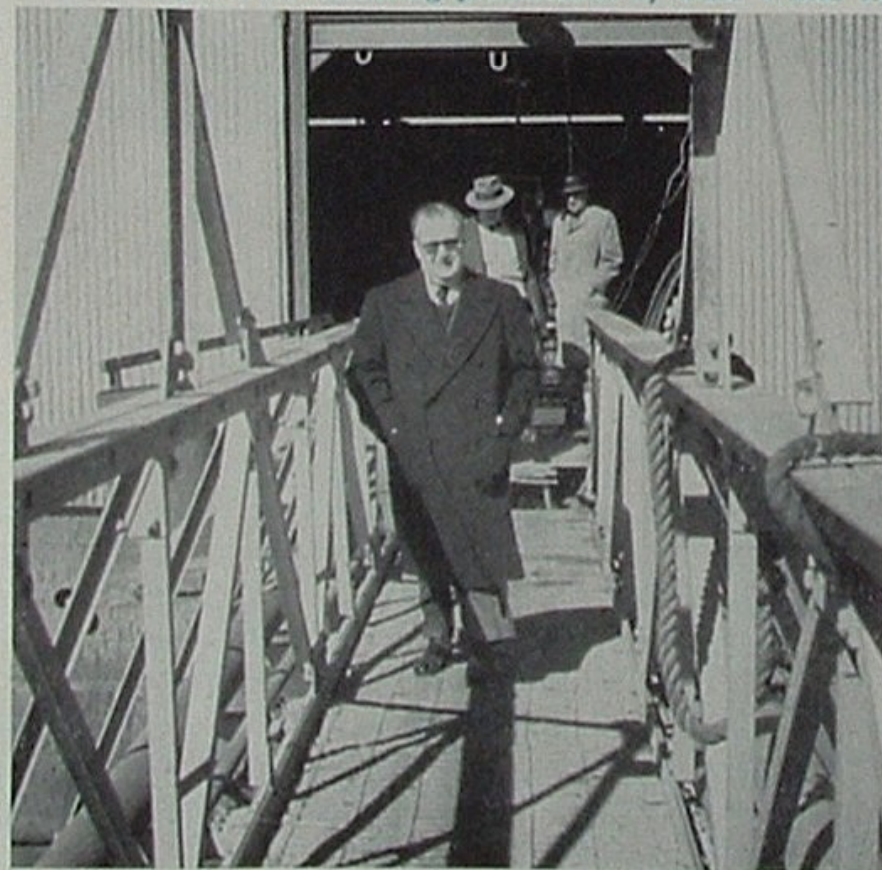
Seen "walking the plank" between drilling and boiler barges of West White Lake drilling rig is Frederic H. Brandt of New York, newest member of Union Oil Board.
