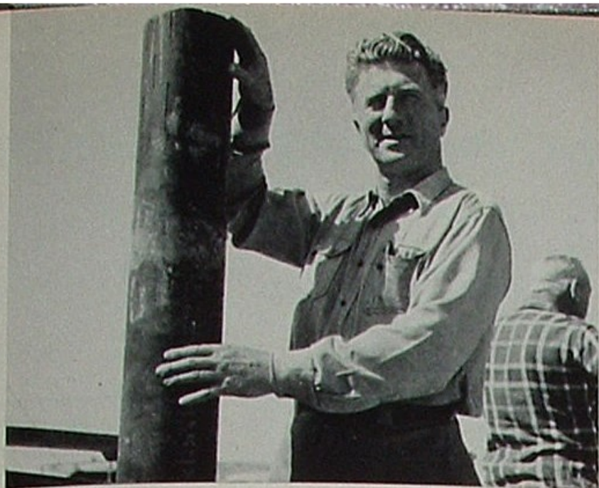
Carl Steiner, division petroleum engineer, indicates with his right hand openings in a section of casing. Such slotted pipe is installed only through layers of productive oil sand.
