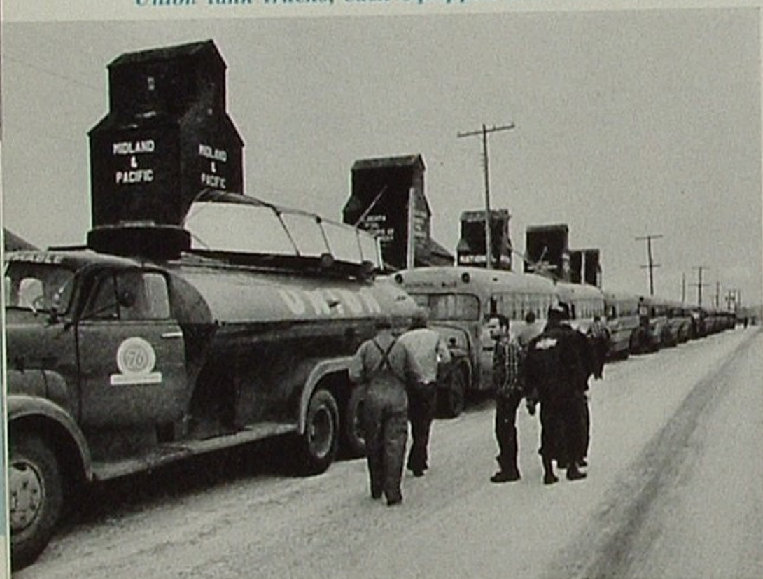
Starting the motors at Whitehorse after a two-day stop required an improvised canvas hood heated underneath with blow torches. The drivers started better on coffee.
