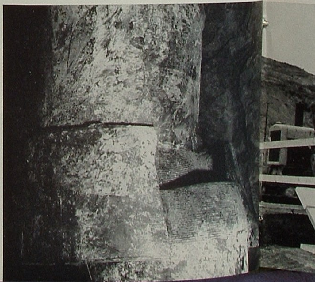
Force of the slowly creeping landslide was so great that the steel collar, right, holding two sections of oil well casing together snapped apart like cardboard.
