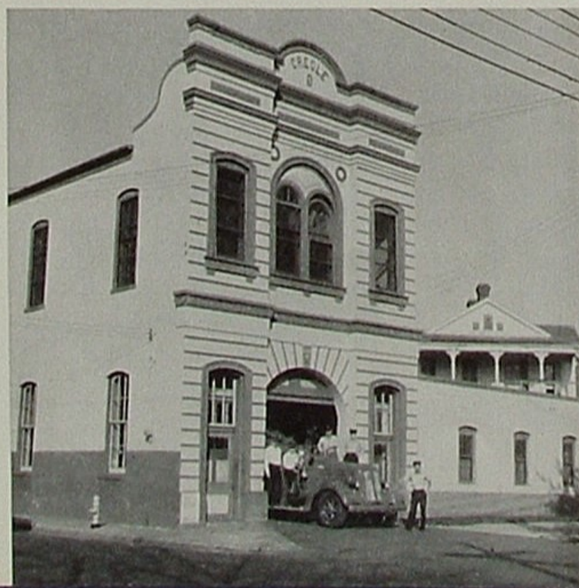
Creole No. 9 Fire Station, at Decatur and Esplanade, stands within a half-block of city's former slave market.
