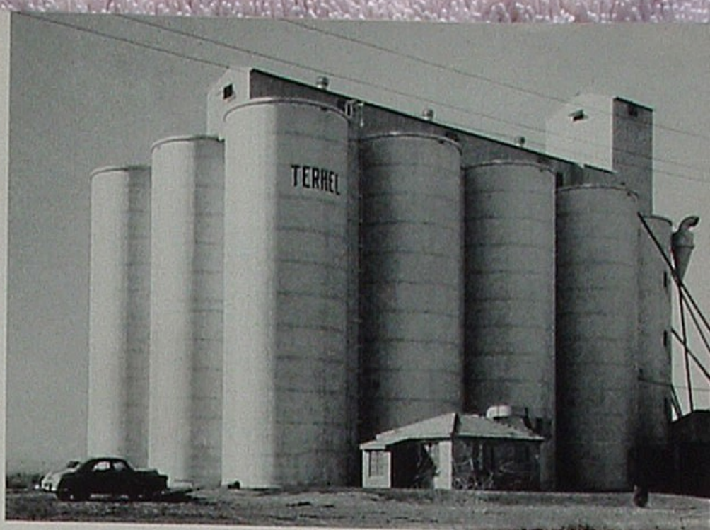
A normally good harvest from surrounding fields will tax the 20-million-pound capacity of these rice tanks. Equipment here consists of scales, mechanical conveyors, driers and blowers. Trucks move the crop to mills during winter.
