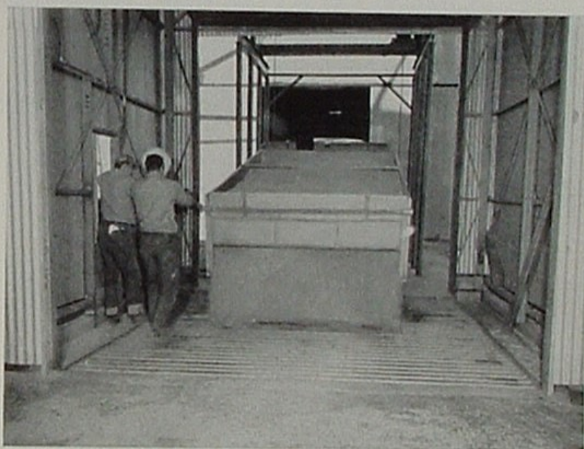
By mechanically lifting the truck's front end, the load is deposited in underground bin of Terhel rice elevator.
