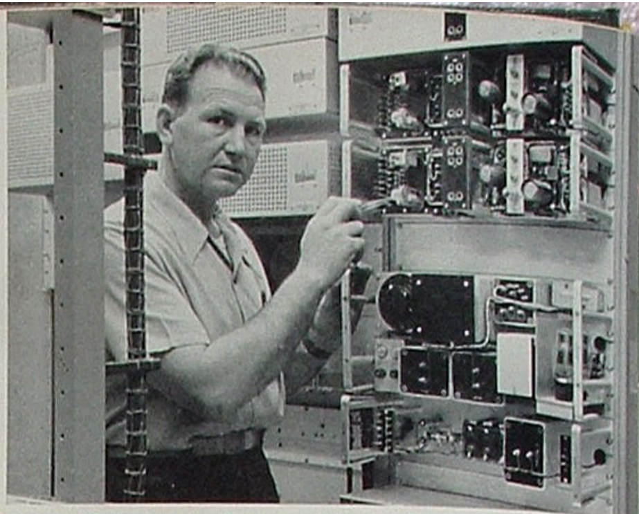
George Robertson points to carrier radio equipment that enables each pair of wires to carry an additional call.
