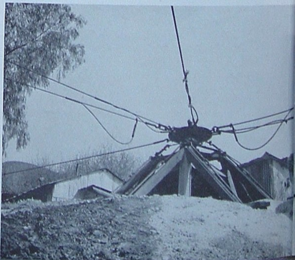
Adams Canyon wells, No. 32 at left, are older than Union Oil Company. Their continued operation is worthwhile only because ancient jack lines, below, endure year after year and permit pumping several wells with one engine.
