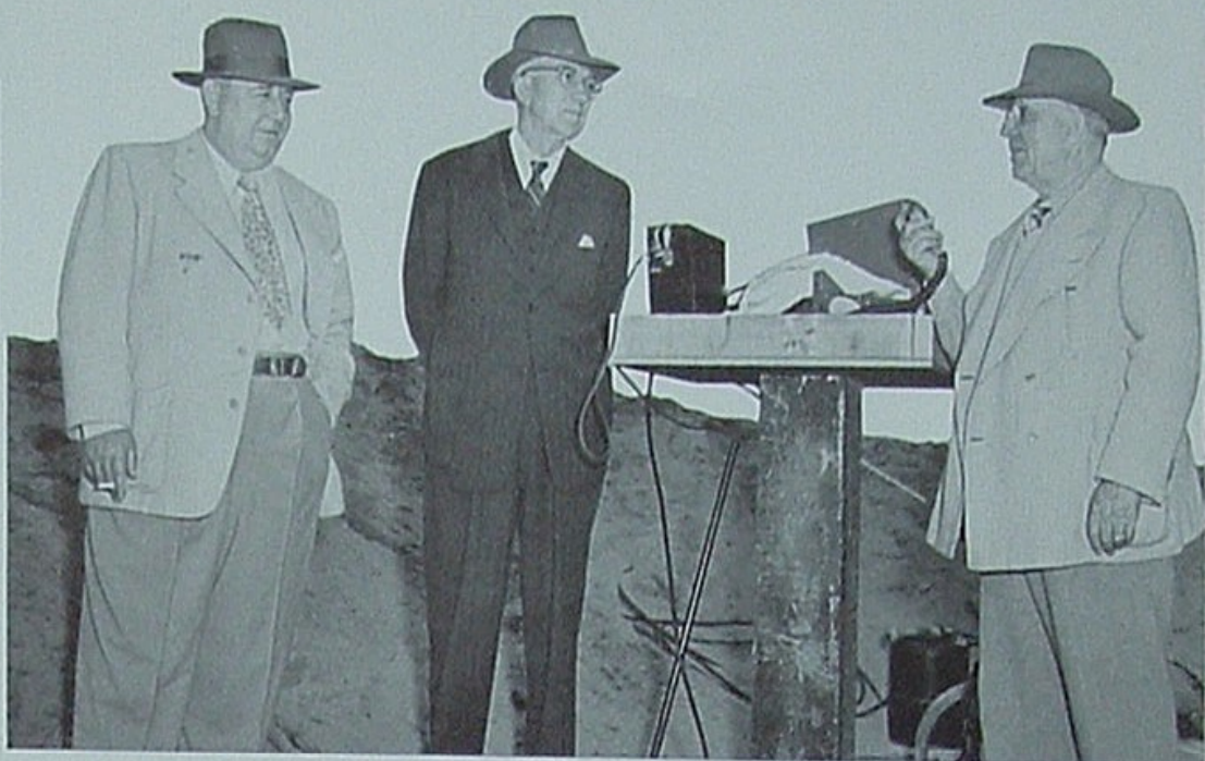
Most pleased with having installed the Pacific Coast's longest submarine oil line are B. L. Haviside, Howard Robinson of Union Oil, and H. T. Haviside, experts all.
