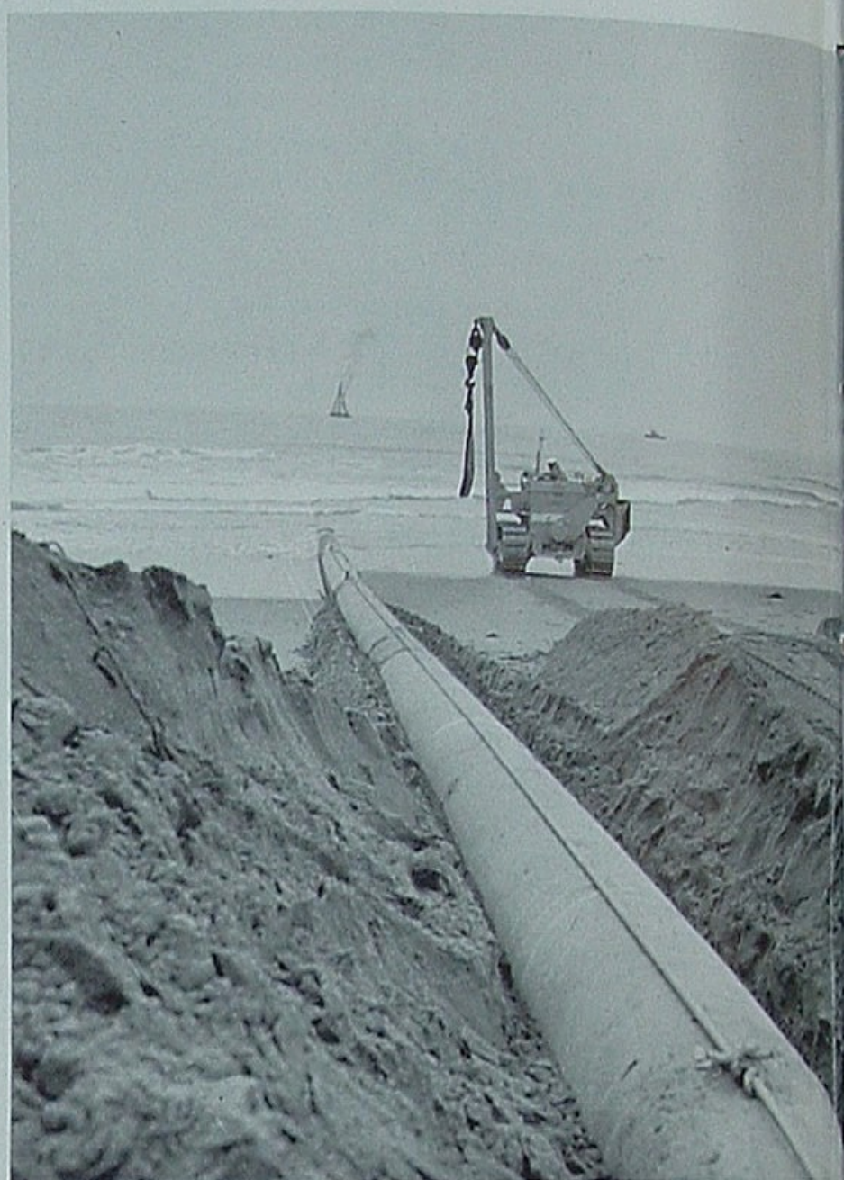
Greatest drag on the pipe occurred across a shoulder of beach where neither rail cars nor water lift could help.
