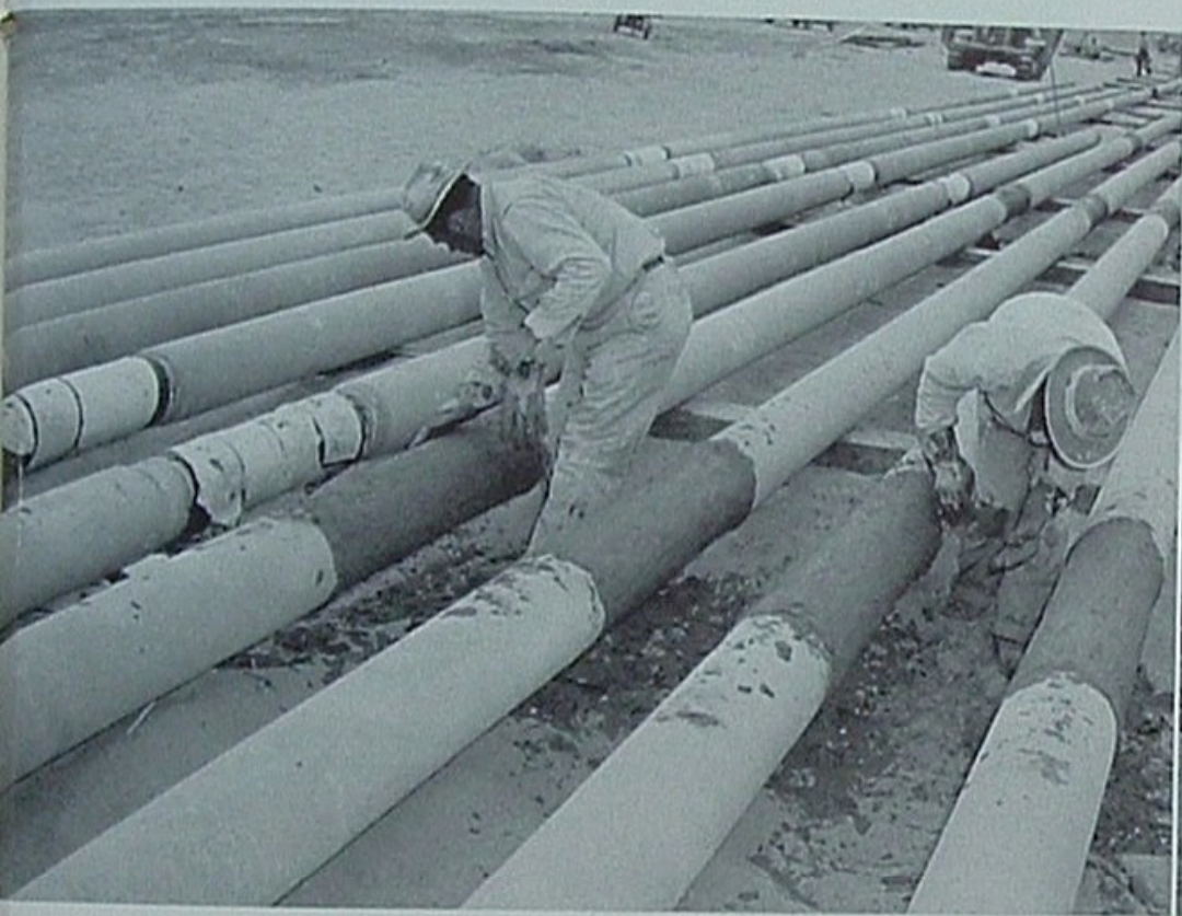
A hand-applied covering of concrete over the final canvas wrap gave the pipe uniform weight and protection.
