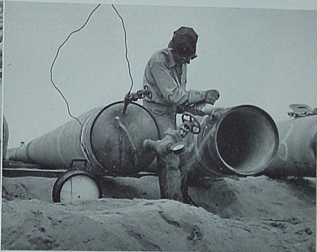
Sealed at both ends, the long pipe sections were subjected to hydrostatic pressure to insure against leaks.
