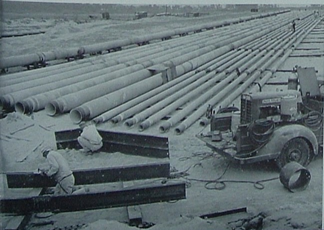
Finally, with 4,800 feet of 20-inch and 4,600 feet of 8-inch line assembled by the ocean . . . . .
