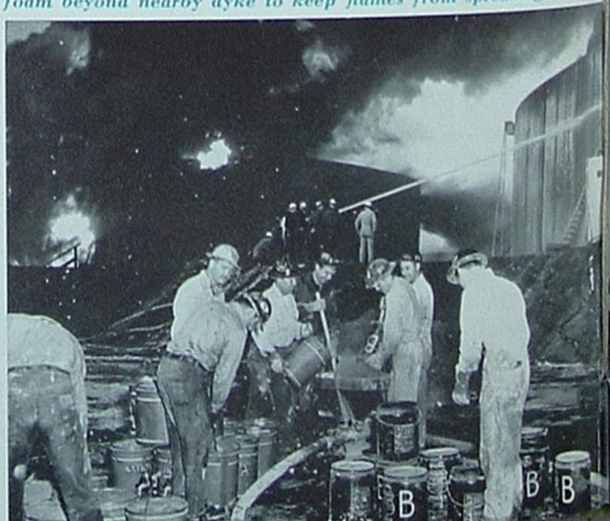
Mixing over 300,000 pounds of foam powders with water, refinery workmen manufactured a lake of fire-smothering foam beyond nearby dyke to keep flames from spreading.
