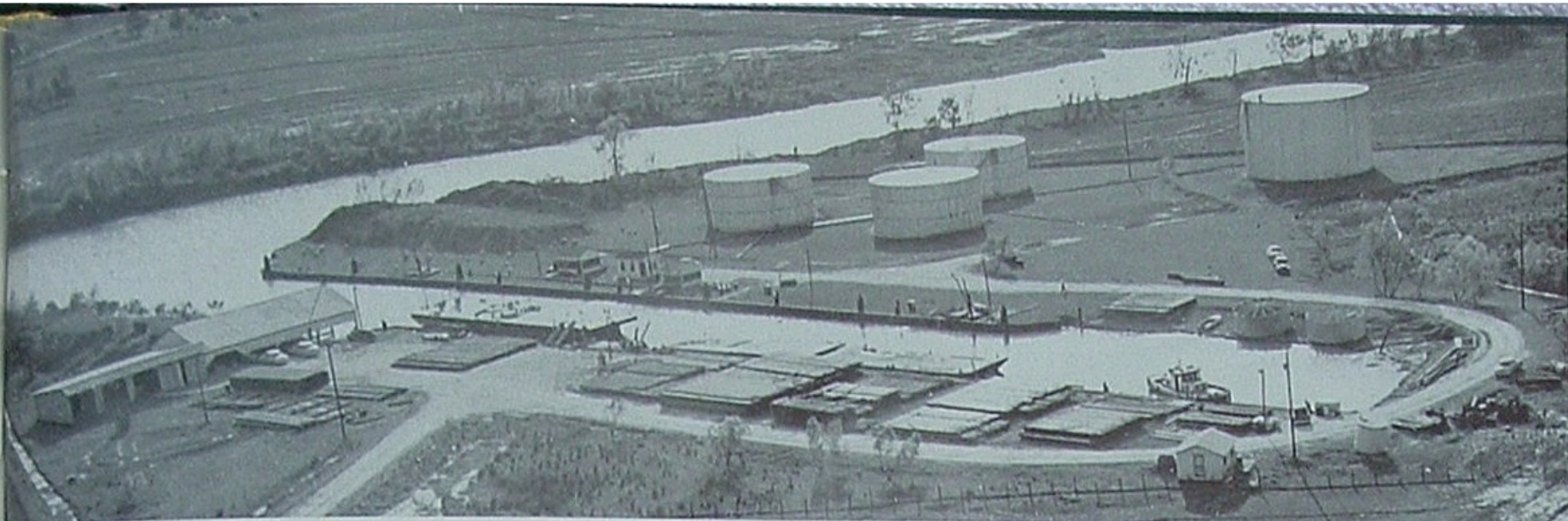
At Forked Island Terminal, crude oil, collected by shallow-draught barges from Union Oil wells in surrounding lakes and marshes, is transferred to larger barges for transportation via the Intracoastal Canal to refineries along Gulf of Mexico.
