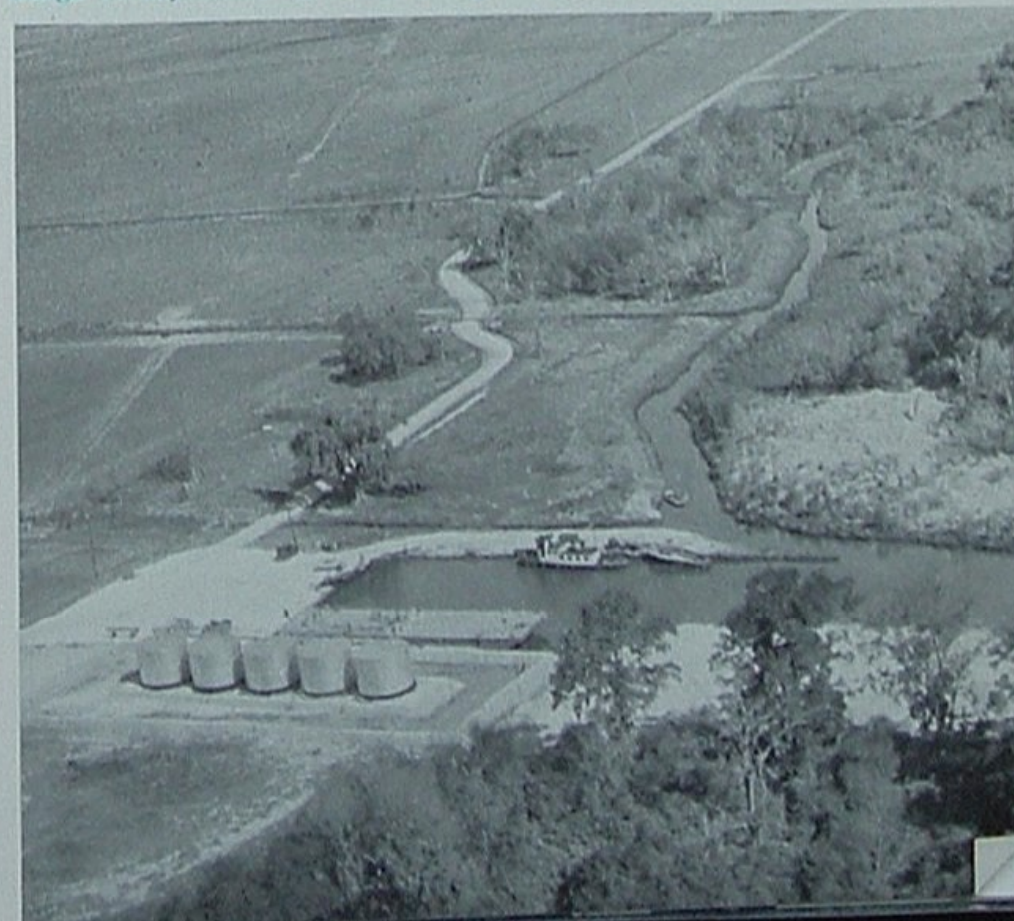
Our present 19 Tigre Lagoon wells produce 40 million cubic feet of gas and 2,000 barrels of distillate and black oil daily. The installations above separate free water and distillate from the natural gas, which gas is then dispatched toward New York via Transcontinental Pipe Line. Black oil and distillate, gathered in tanks below, are sent by barge to refineries of other companies via Forked Island.
