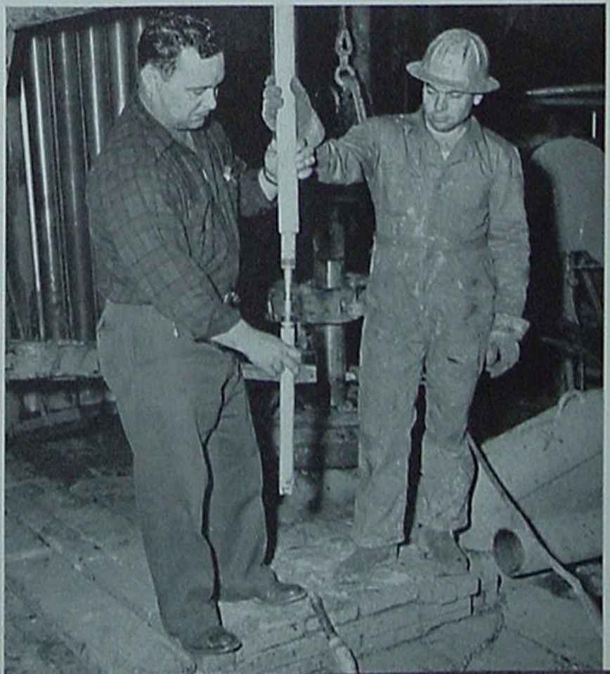
. . . . . and connecting a flashlamp to provide light, and finally loading the device to make a compass reading.
