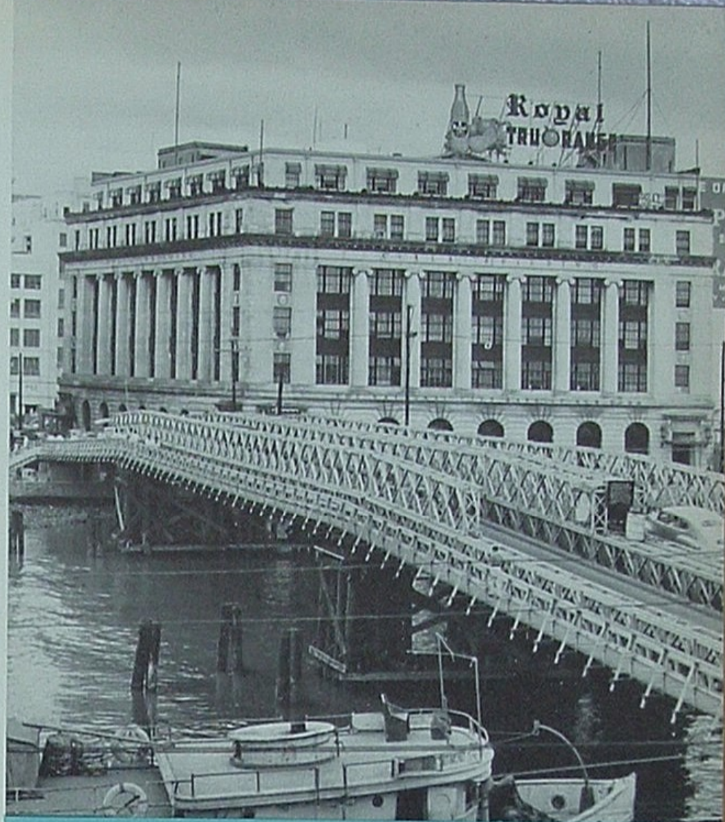
A temporary Bailey bridge leads to Theo. H. Davies & Co., Far East, Ltd., Ayala Building offices in Manila.
