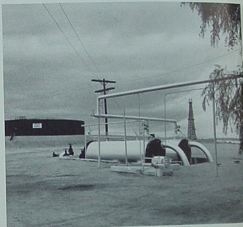
Below, Glenn Woods, district foreman, presses the button starting fire in the boilers. Resulting steam flows to heat exchangers, above, heating crude oil to 160 degrees.
