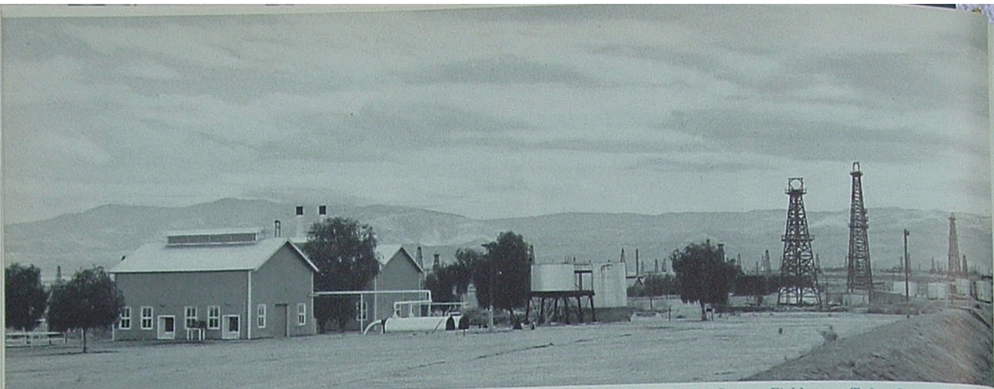
Operating entirely without human attendance is this Union Oil pump station in the Sunset Field near Taft. Originally built in 1909, close to famous Lake View No. 1, it now boasts automatic boilers and self-driven engines and pumps.
