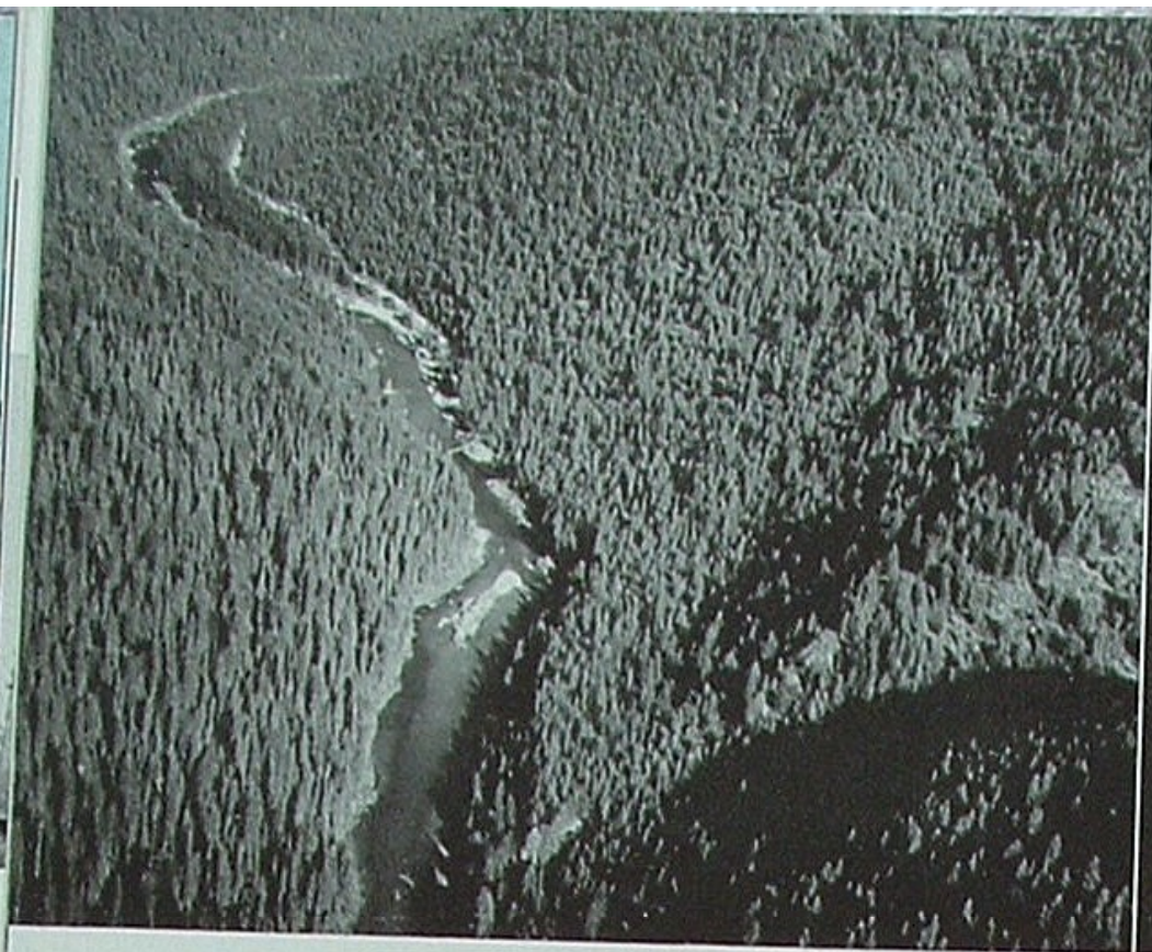
The reservoir area of Hungry Horse Dam looked forbidding to land-clearing contractors as they flew over it in 1948 and envisaged the enormous tree-cutting job that lay ahead.
